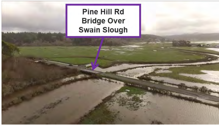
Figure 5. Flooding During a Severe Storm Event in 2017 (view of the bridge from the northwest looking southeast; photograph provided as part of the 2019 Agricultural Suitability Assessment prepared by Stantec).
