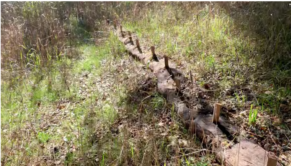
Weak mitigation measure with straw-burlap wattles above the collapsing bank of Olema Creek, and seeded non-native grains. January 26, 2020. Photo: Laura Cunningham.
