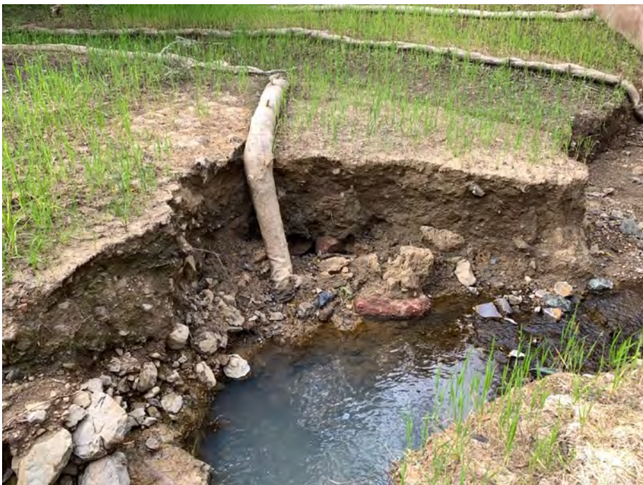
Olema Creek critical habitat for salmonids in very poor condition from chronic cattle grazing in the watershed. Streambank collapse causes sedimentation of salmon spawning gravels and poor water quality. Mitigation baffles are also collapsing into the eroding and unstable streambank and are ineffective. Golden Gate National Recreation Area. April 15, 2019. Photo: Laura Cunningham.
