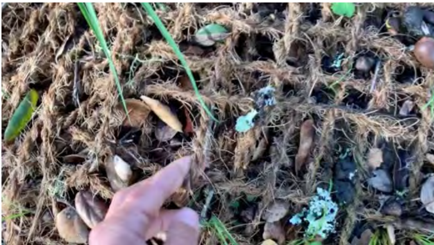
Weak mitigation measure of aging fiber netting placed across highly-eroded and trampled cattle path that formerly crossed Olema Creek. January 26, 2020. Photo: Laura Cunningham.
