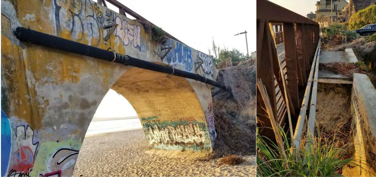
**Figure 7.** Existing infrastructure (sewer main and PG&E electrical conduit) located on pedestrian bridge and cement arch bridge.
