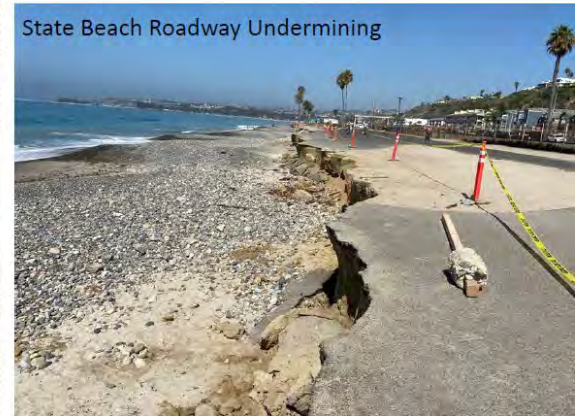
FIGURE 2-3. NORTH REACH – UNDERMINING OF ASPHALT AND ERODED BEACH CONDITIONS
