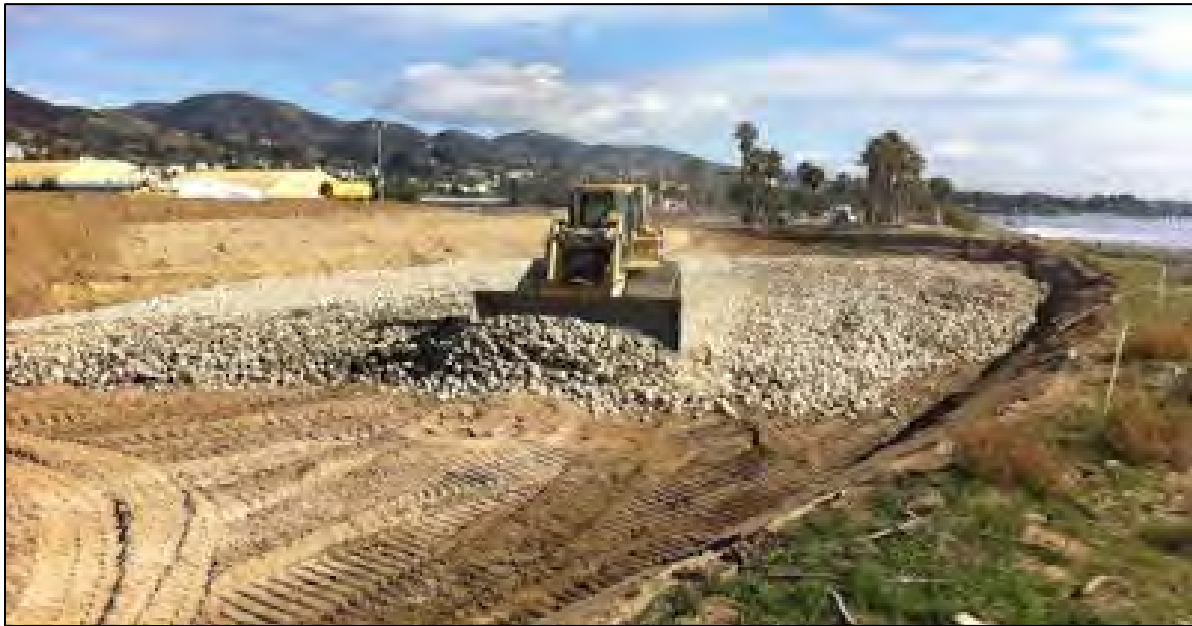
FIGURE 3-6. CONSTRUCTION OF A COBBLE BERM AT SURFER'S POINT
