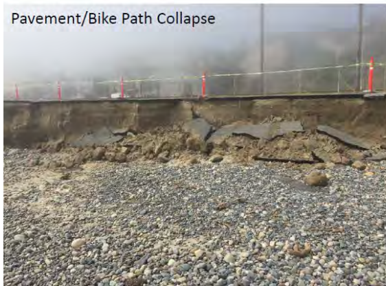
FIGURE 2-3. NORTH REACH – UNDERMINING OF ASPHALT AND ERODED BEACH CONDITIONS
