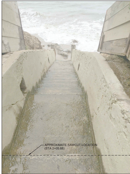
1 SAW CUT APPROXIMATE LOCATION D-501 SCALE: NONE
