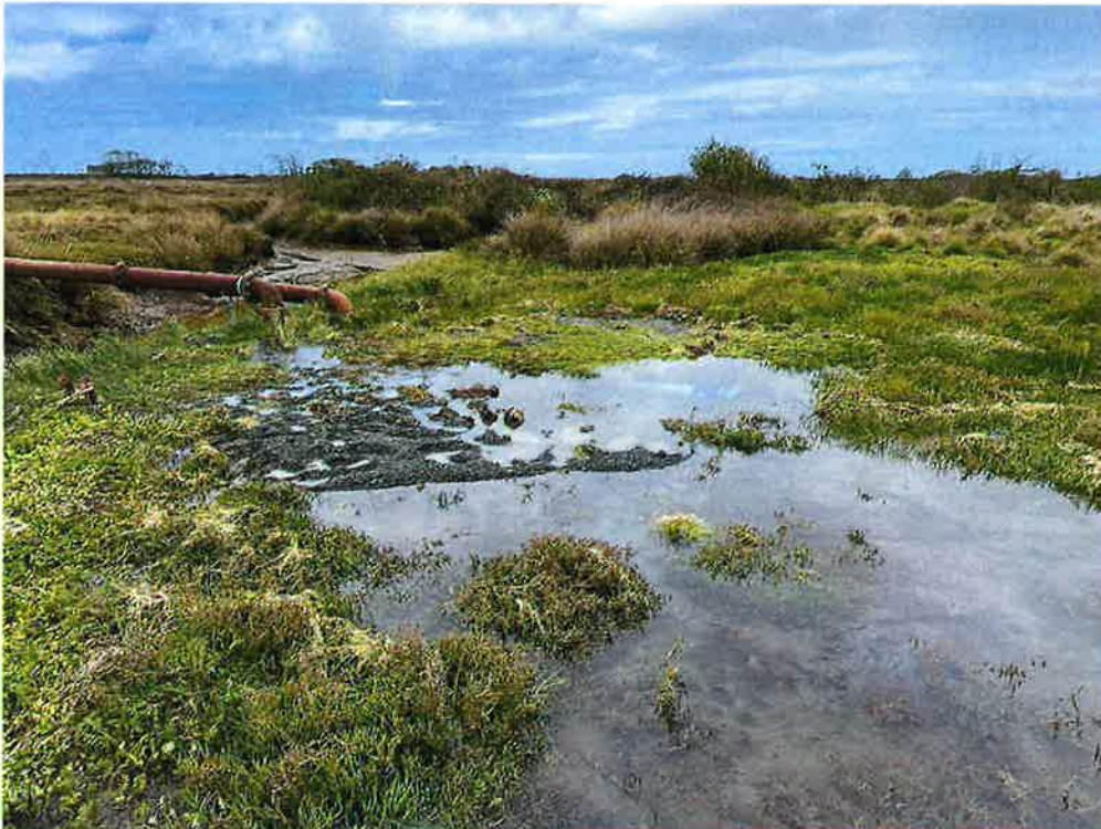
4/19/22 – Emergency Repair Location – See displaced gravel
