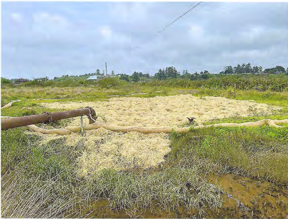
4/25/22 – Emergency repair site #1 completed
