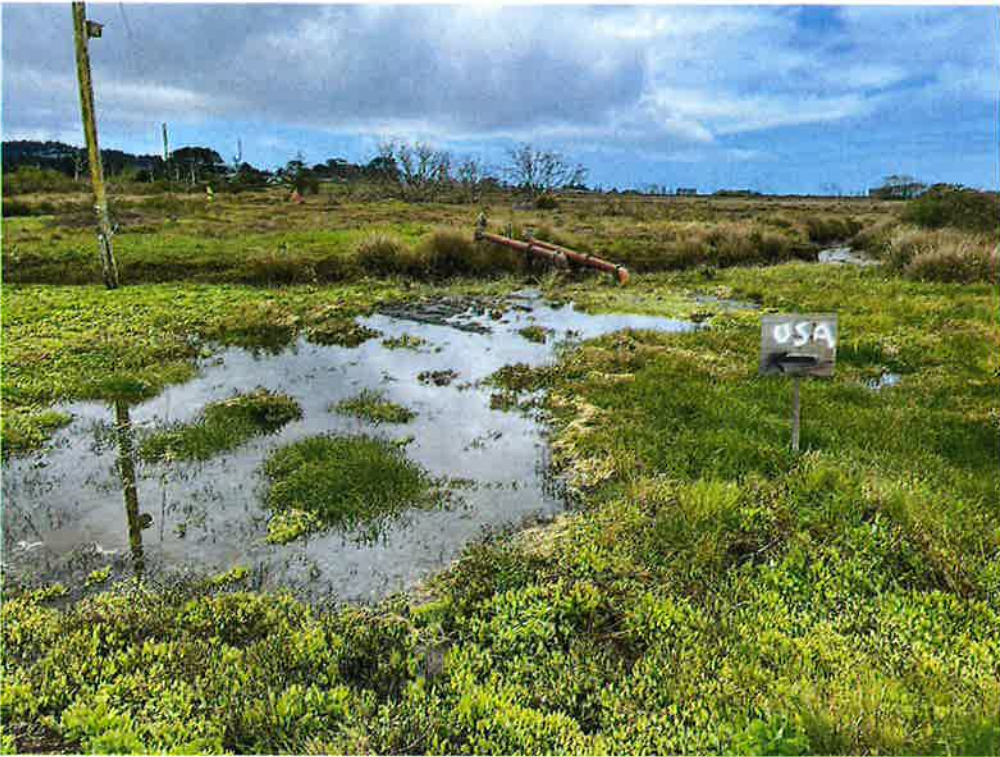
4/19/22 – Emergency Repair Location - Overview
