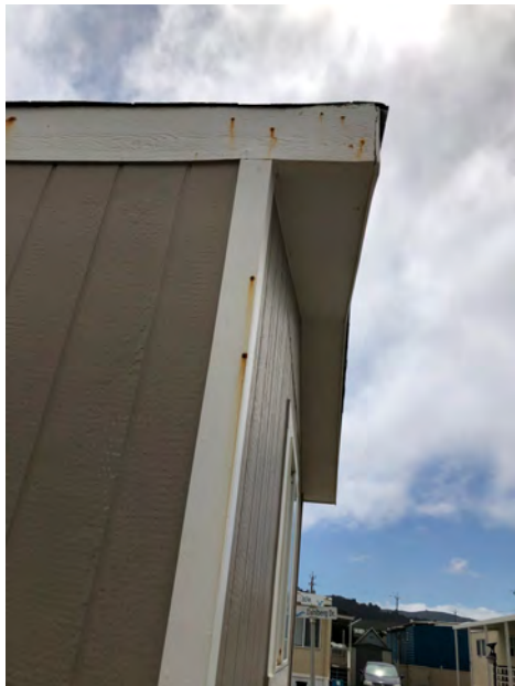
200 Second Ave - Fascia detail at roof. Fascia typical of original construction. Evidence of fascia wear and indications of maintenance, including re-painting. No evidence of any modifications to structural roof or wall elements. Roof replacement likely would have included overhang
