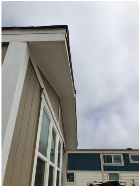
332 Third Ave - Fascia detail at roof reflecting non-structural repair and maintenance, including re-painting. Fascia typical of original construction. If roof structural framing had been replaced, boxed eave and fascia would not show similar wear. Replacement of roof elements likely would have included overhang. No evidence of modifications to structural roof elements.
