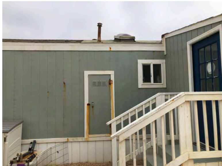
412 Fourth Ave - Side view, entry steps. Gable roof, no overhang. T1-11 siding typical of original construction. No indication that removal or replacement of structural wall framing has occurred.
