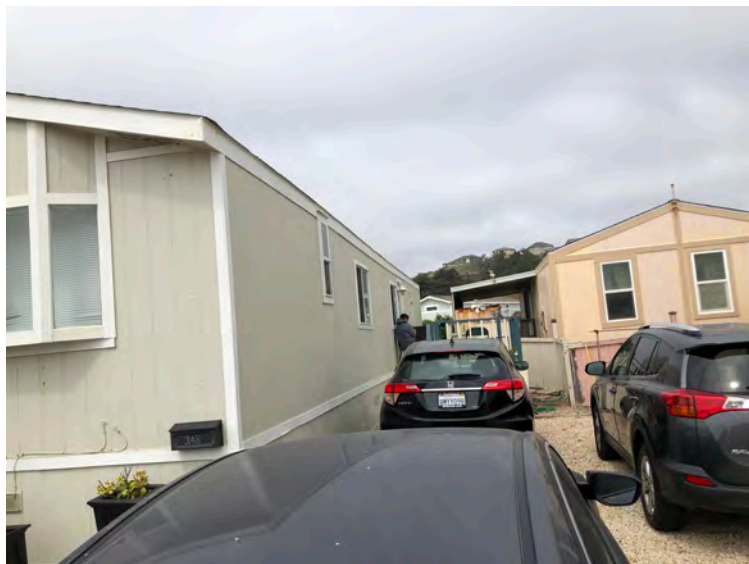
348 Third Ave - Side view. Gable roof, no overhang. T1-11 siding typical of original construction. No indication that removal or replacement of structural wall framing has occurred.
