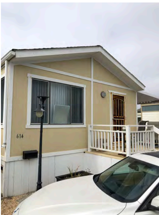
614 Sixth Ave - Front elevation. Gable roof with no overhang, typical of original construction. If roof framing had been replaced, likely would have been built with an overhang.
