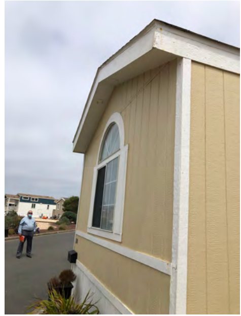
204 Second Ave - Fascia detail at roof. If roof structural framing had been replaced, boxed eave and fascia would not show similar wear. Replacement of roof elements likely would have included overhang.
