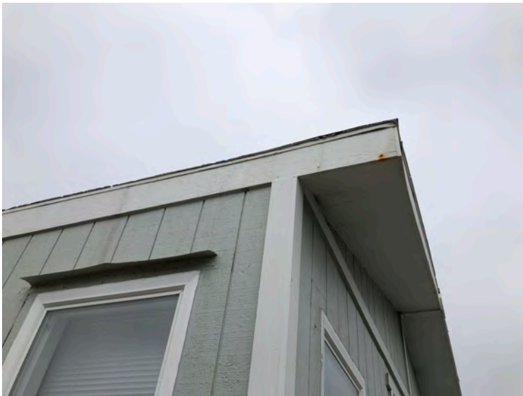
149 First Ave - Left side. No overhang. Evidence of prior window replacement without modification of structural wall elements. T1-11 siding typical of original wall covering.
