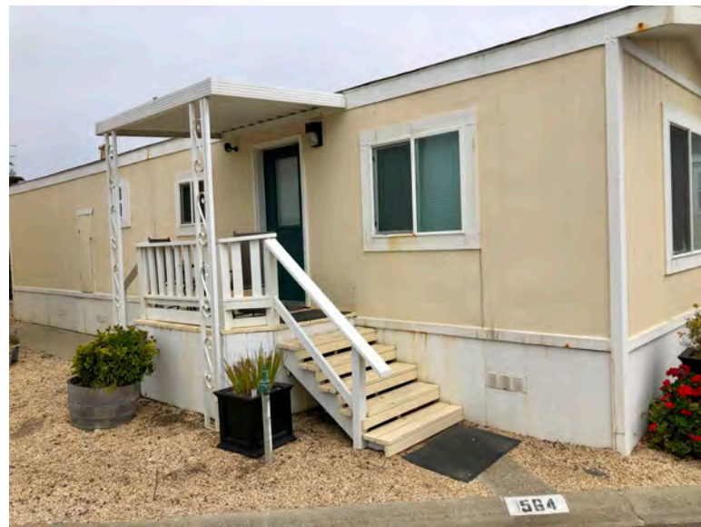
564 Fifth Ave - Materials and gable roof with little or no overhang typical of original construction. No indication that removal or replacement of structural roofing has occurred. Replacement would have had significant impact on wall framing and interiors and likely would have been built with an overhang.
