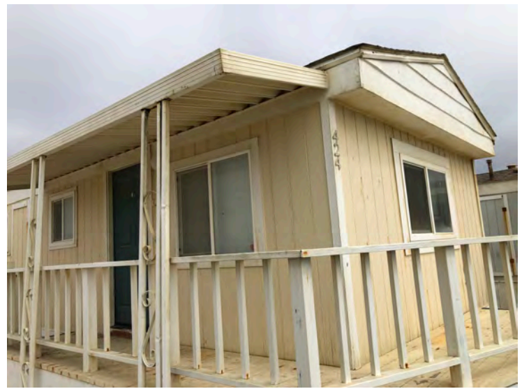
424 Fourth Ave - Materials and gable roof with little or no overhang typical of original construction. No indication that removal or replacement of structural roofing has occurred. Replacement would have had significant impact on wall framing and interiors and likely would have been built with an overhang.
