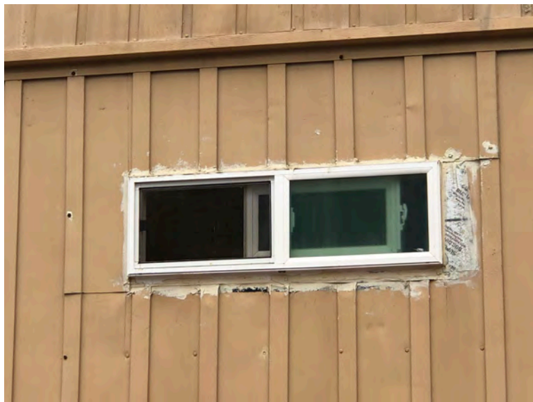
622 Sixth Ave - Side wall elevation. Small window appears to have been inserted into original metal wall covering. Window is smaller in size than other windows and appears to have been added later in time. Evidence of patch and repair of surrounding wall covering area.
