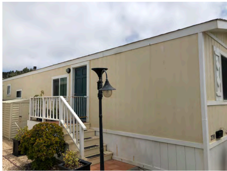
220 Second Ave - Side view with T1-11 siding. Evidence of non-structural repair and maintenance (e.g. caulking, sealing) of T1-11 wall covering. T1-11 siding typical of original construction. No indication that any removal or replacement of structural wall framing has occurred.
