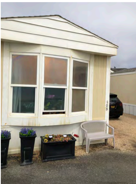
408 Fourth Ave - Front elevation. Gable roof with no overhang, pop out window, typical of original construction. If roof framing had been replaced, likely would have been built with an overhang.
