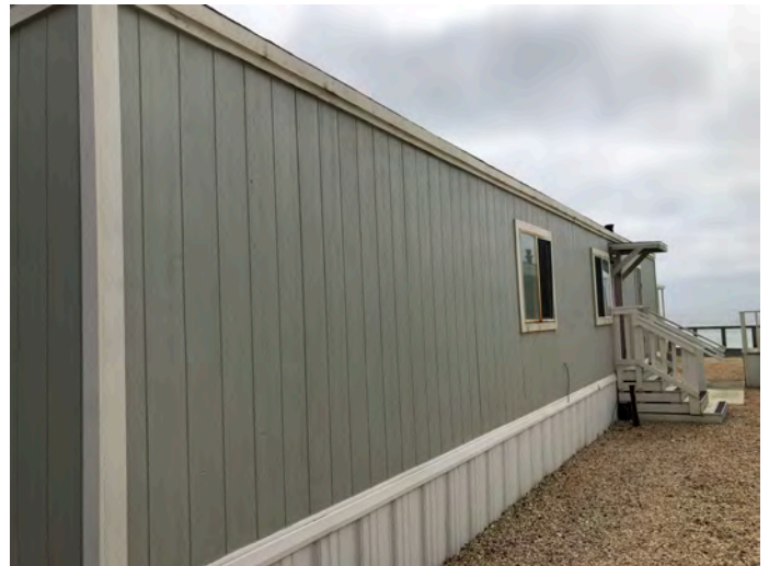
345 Third Ave - Exterior T1-11 siding wall covering. Evidence of non-structural repair and maintenance (e.g., caulking, sealing) of T1-11 wall covering. T1-11 siding typical of original construction. No indication that removal or replacement of structural wall framing has occurred.
