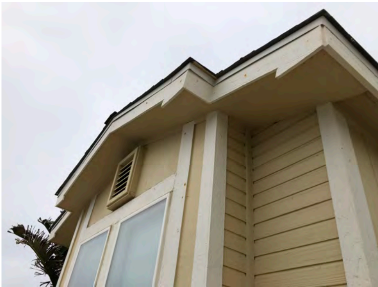
580 Fifth Ave - Front elevation with boxed eave and pop out window bay typical of original construction. No indication of modifications to structural roof elements.
