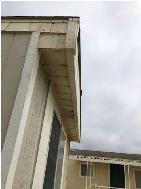
428 Fourth Ave - Gable roof, no overhang. T1-11 siding and fascia typical of original construction. Fascia wear at roof. If roof structural framing had been replaced, fascia would not show similar wear. Replacement of roof elements likely would have included overhang.
