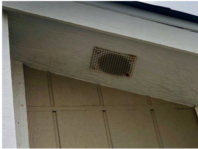
317 Third Ave - Fascia detail at roof with boxed eave, no overhang. Note old style vent at boxed eave, typical of original construction.
