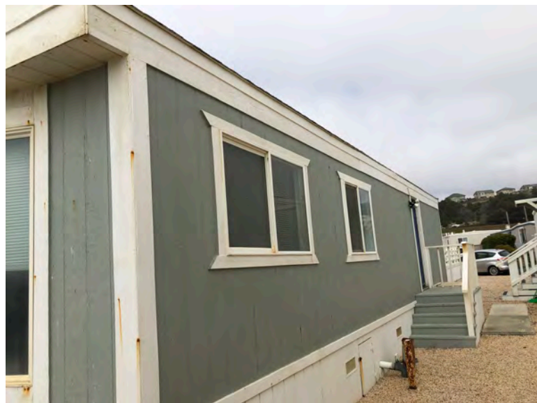
444 Fourth Ave - T1-11 siding typical of original construction. Fascia wear at roof. If roof structural framing had been replaced, fascia would not show similar wear. Replacement of roof elements likely would have included overhang. Evidence of patch and repair of wall surface without modification of structural elements.
