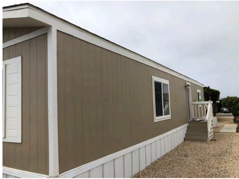
157 First Ave - Right side elevation. T1-11 siding typical of original wall covering. Gable roof construction, no overhang. Typical of original unit.
