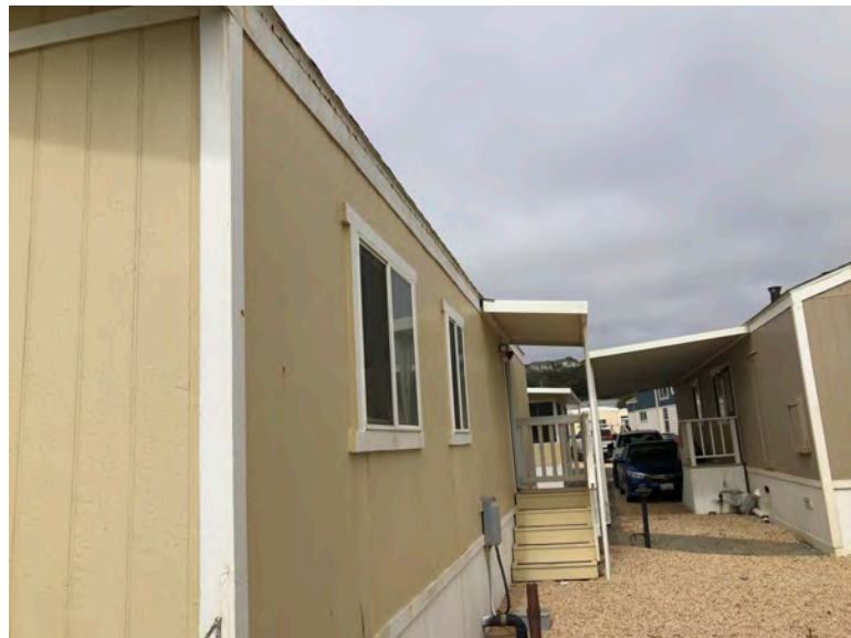
416 Fourth Ave - Side elevation, entry steps. Gable roof, no overhang. T1-11 siding typical of original construction. No indication that any removal or replacement of structural wall framing has occurred.
