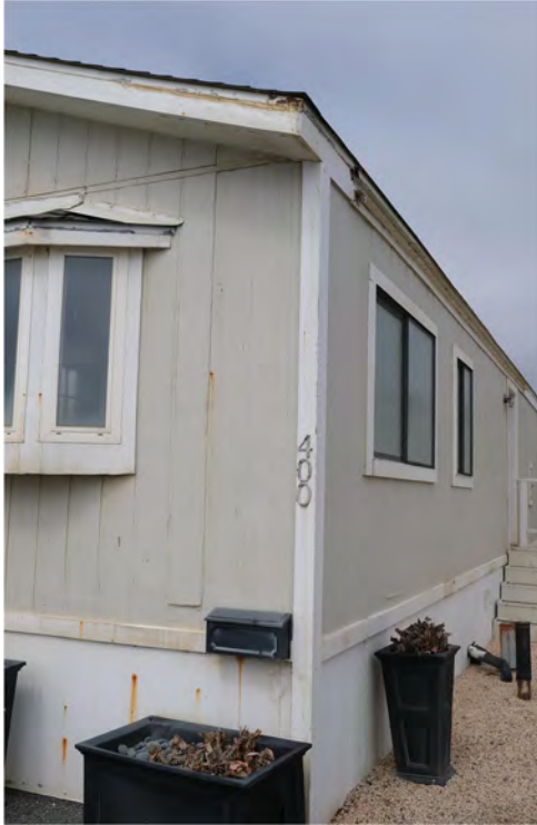
400 Fourth Ave - Front elevation. Gable roof with no overhang, pop out window, typical of original construction. If roof framing had been replaced, likely would have been built with an overhang.
