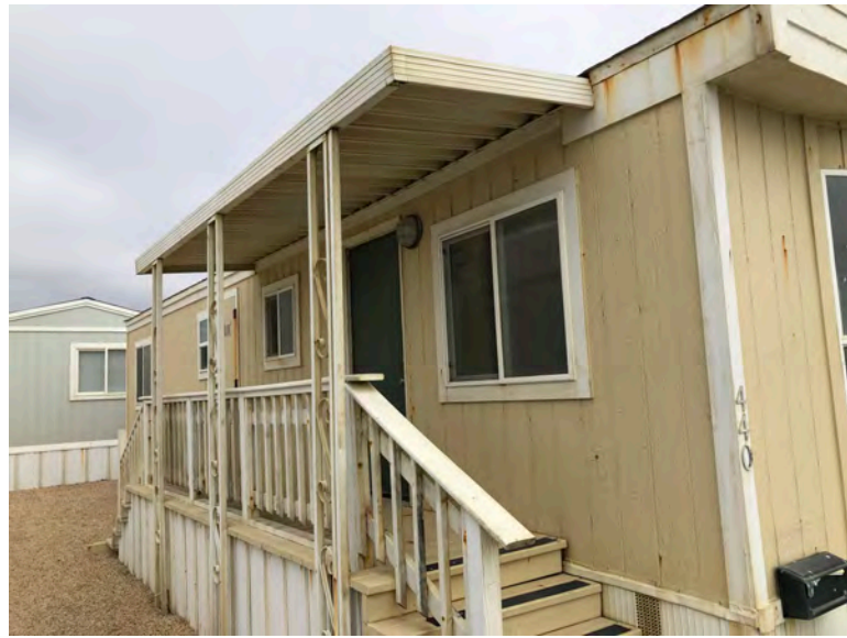
440 Fourth Ave - Side view, entry steps. T1-11 siding and fascia typical of original construction. Fascia wear at roof. If roof structural framing had been replaced, fascia would not show similar wear. Replacement of roof elements likely would have included overhang.
