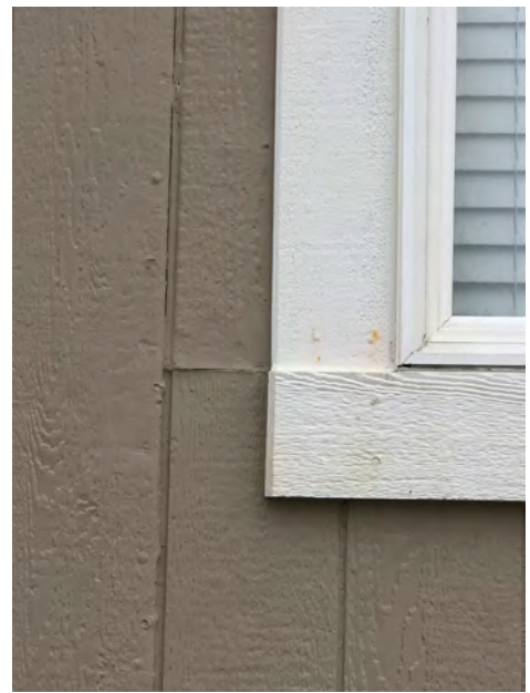
200 Second Ave - Evidence of repair and maintenance (e.g., caulking, sealing) of T1-11 wall covering. No indication that removal or replacement of structural wall framing has occurred.
