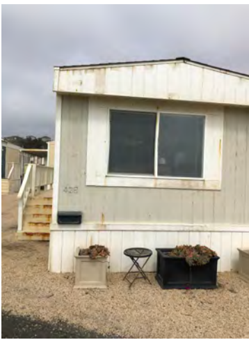
428 Fourth Ave - Front elevation with side entrance ("shotgun installation"). Gable roof with no overhang typical of original unit. No evidence of any modifications to structural roof elements. Roof replacement would have had significant impact on wall framing and interiors and likely would have included a roof overhang.
