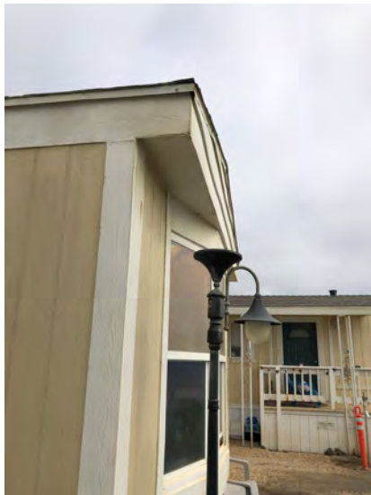
408 Fourth Ave - Gable roof, no overhang. T1-11 siding typical of original construction. Fascia wear at roof. If roof structural framing had been replaced, boxed eave and fascia would not show similar wear. Replacement of roof elements likely would have included overhang.
