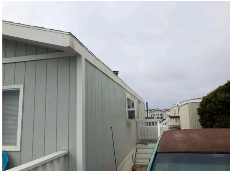
149 First Ave - Right side elevation. T1-11 wall covering with gable roof and no overhang. No indication of modifications to structural roof or wall elements.
