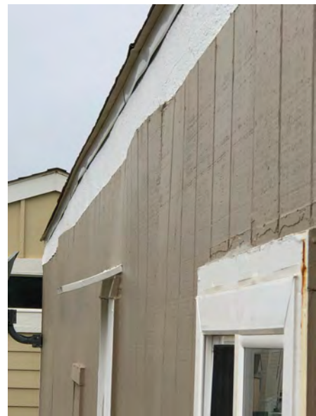
157 First Ave - Side elevation. Evidence of prior window replacement without modification of structural wall elements. Evidence of non-structural repair and maintenance (e.g., caulking, sealing) of T1-11 wall covering. T1-11 siding typical of original construction. No indication that any removal or replacement of structural wall framing has occurred.
