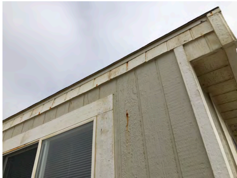
428 Fourth Ave - Side elevation. Gable roof, no overhang. T1-11 siding typical of original construction. No indication that removal or replacement of structural wall framing has occurred.
