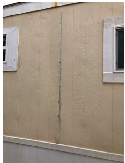
564 Fifth Ave - Existing T1-11 siding reflecting wear and non-structural repair and maintenance. If structural wall framing had been replaced, siding would not show similar wear.
