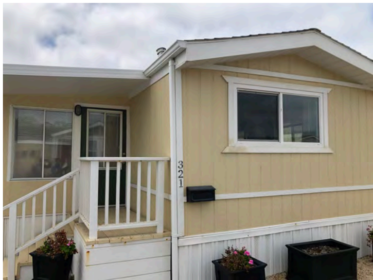
321 Third Ave - Front elevation. Gable roof with no overhang, typical of original construction. Replacement would have had significant impact on framing and interiors and likely would have been constructed with an overhang.
