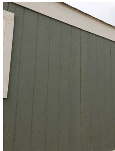
436 Fourth Ave - Side elevation. Gable roof, no overhang. T1-11 siding typical of original construction. Evidence of patch and repair of wall surface. No indication that removal or replacement of structural wall framing has occurred.
