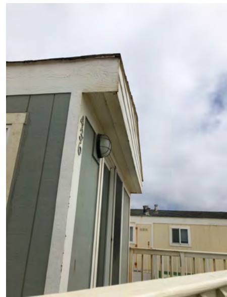
436 Fourth Ave - T1-11 siding and fascia typical of original construction. Fascia wear at roof. If roof structural framing had been replaced, fascia would not show similar wear. Replacement of roof elements likely would have included overhang.
