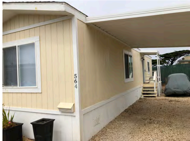
564 Fifth Ave - Side elevation. Gable roof, no overhang. T1-11 siding typical of original construction. No indication that removal or replacement of structural wall framing has occurred.
