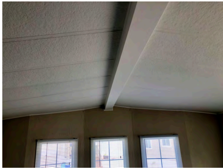
325 Third Ave - Interior elevation of open ceiling with boxed beam, indicative of original gable construction. Interior finish materials at ceiling consistent with type used in older models of this genre.
