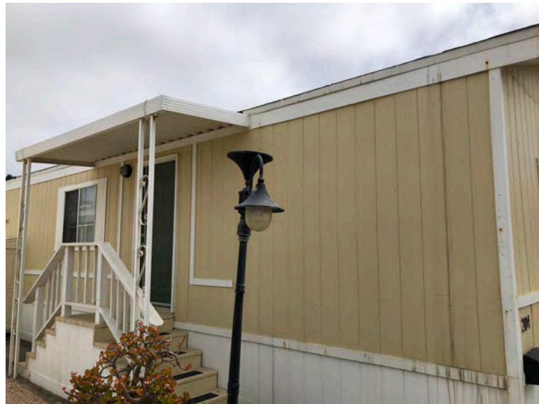
204 Second Ave - Side view with T1-11 siding. Evidence of non-structural repair and maintenance (e.g., caulking, sealing) of T1-11 wall covering. No indication that removal or replacement of structural wall framing has occurred.
