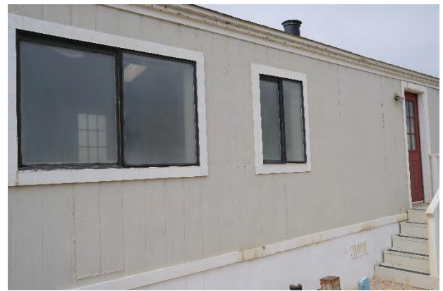
400 Fourth Ave - Side view, entry steps. Gable roof, no overhang. T1-11 siding typical of original construction. No indication that removal or replacement of structural wall framing has occurred.
