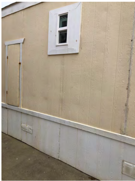
564 Fifth Ave - Existing T1-11 siding reflecting wear, evidence of patch and repair without modification of structural elements. If structural wall framing had been replaced, siding would not show similar wear.
