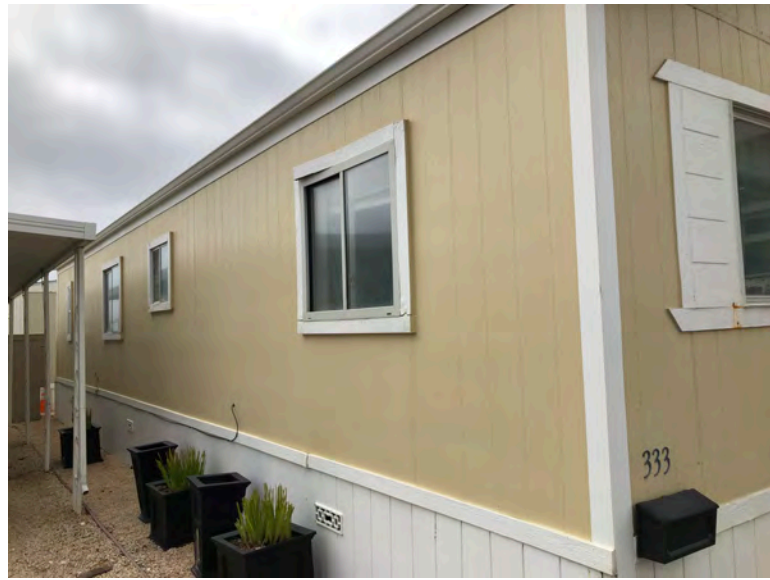
333 Third Ave - Side view, no overhang. Side view with T1-11 siding. Evidence of non-structural repair and maintenance (e.g., caulking, sealing) of T1-11 wall covering. T1-11 siding typical of original construction. No indication that removal or replacement of structural wall framing has occurred.
