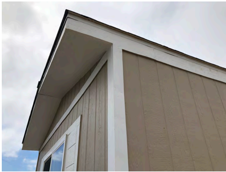
157 First Ave - Front elevation with boxed overhang at front gable. Typical of original construction. No evidence of removal or replacement of structural roof framing system or wall elements.
