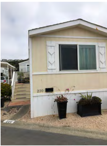
220 Second Ave - Front Elevation with side entrance ("shotgun installation"). Materials and gable roof with little or no overhang typical of original construction. No indication that removal or replacement of structural roof framing has occurred. Replacement would have had significant impact on wall framing and interiors and likely would have been constructed with an overhang.
