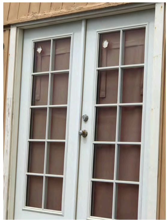
622 Sixth Ave - Side wall elevation showing door that appears to have been inserted into area previously occupied by a window. Non-load bearing portion of wall previously located below window appears to have been removed to allow for the door. Addition of door should not have resulted in alteration of structural wall elements.
