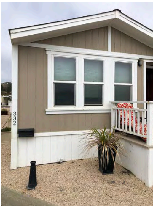
332 Third Ave - Front Elevation. Gable roof with no overhang, typical of original construction. If roof framing had been replaced, likely would have been constructed with an overhang.
