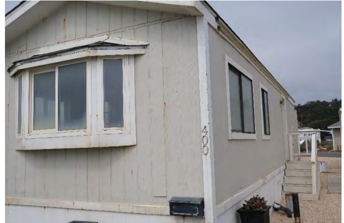
400 Fourth Ave - Side view, entry steps. Materials and gable roof with little or no overhang typical of original construction. No indication that removal or replacement of structural roofing has occurred. Replacement would have had significant impact on wall framing and interiors and likely would have been built with an overhang.
