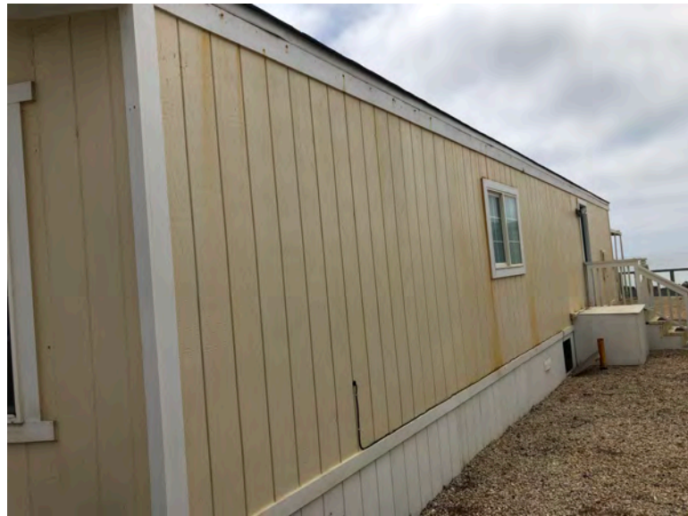
325 Third Ave - Side view with T1-11 siding. Evidence of non-structural repair and maintenance (e.g., caulking, sealing) of T1-11 wall covering. T1-11 siding typical of original construction. No indication that any removal or replacement of structural wall framing has occurred.
