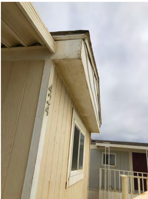
424 Fourth Ave - Gable roof, no overhang. T1-11 siding and fascia typical of original construction. Fascia wear at roof and indications of repair and maintenance. If roof structural framing had been replaced, fascia would not show similar wear. Replacement of roof elements likely would have included overhang.
