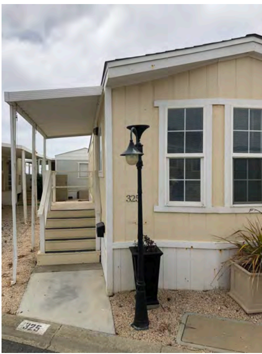
325 Third Ave - Gable roof with no overhang, typical of original construction. Replacement likely would have been constructed with an overhang.
