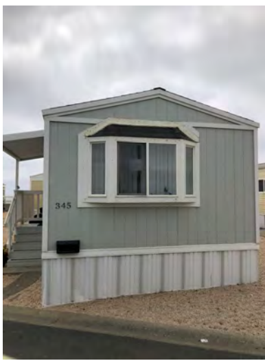
345 Third Ave - Front elevation. Gable roof construction with boxed eave and pop out window, typical of original construction. No indication that removal or replacement of structural roof framing has occurred. Replacement would have had significant impact on wall framing and interiors and likely would have been constructed with an overhang.
