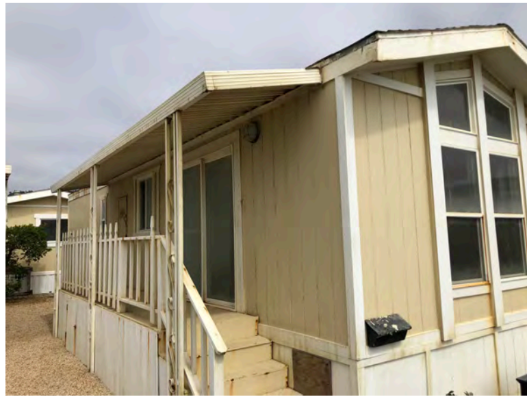
416 Fourth Ave - Side view. T1-11 siding typical of original construction. Fascia wear at roof. If roof structural framing had been replaced, fascia would not show similar wear. Replacement of roof elements likely would have included overhang.
