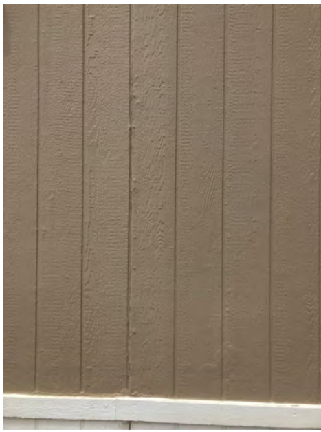
317 Third Ave - Evidence of non-structural repair and maintenance (e.g., caulking, sealing) of T1-11 wall covering. No indication that any removal or replacement of structural wall framing has occurred. If wall framing had been replaced, siding would not show similar wear.
