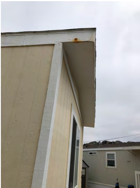
564 Fifth Ave - Gable roof, no overhang. T1-11 siding and fascia typical of original construction. Fascia wear at roof. If roof structural framing had been replaced, fascia would not show similar wear. Replacement of roof elements likely would have included overhang.
