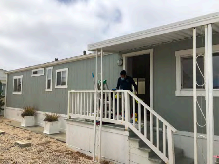
329 Third Ave - Side view. Entry steps. Gable roof, no overhang. T1-11 siding typical of original construction. Evidence of patch and repair of existing T1-11 wall covering. No indication that removal or replacement of structural wall framing has occurred.
