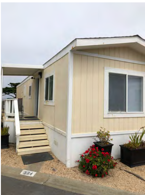
564 Fifth Ave - Front elevation. Gable roof with no overhang, typical of original construction. If roof framing had been replaced, likely would have been built with an overhang.
