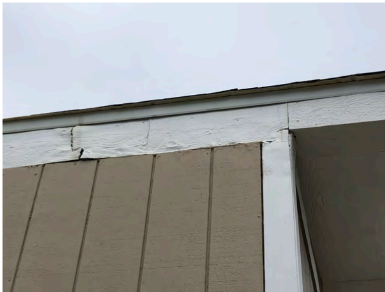
157 First Ave - Fascia typical of original construction. Evidence of fascia wear and indications of maintenance, including caulking and re-painting. No evidence of any modifications to structural roof or wall elements. Roof replacement likely would have included overhang.
