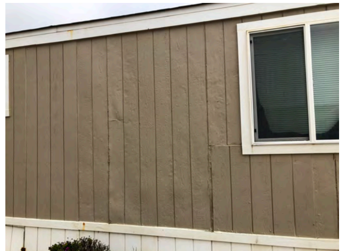
332 Third Ave - Exterior T1-11 siding wall covering. Evidence of non-structural repair and maintenance (e.g., caulking, sealing) of T1-11 wall covering. T1-11 siding typical of original construction. No indication that removal or replacement of structural wall framing has occurred.
