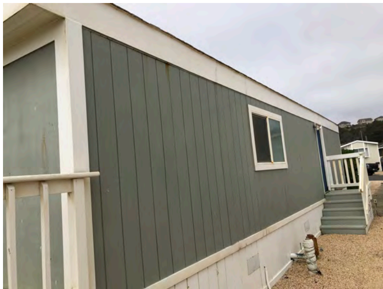
436 Fourth Ave - Side elevation. T1-11 siding typical of original construction. Fascia wear at roof reflecting original construction. If roof structural framing had been replaced, fascia would not show similar wear. Replacement of roof elements likely would have included overhang.
