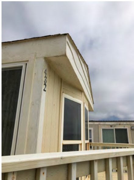
432 Fourth Ave - Gable roof, no overhang. T1-11 siding and fascia typical of original construction. Fascia wear at roof and indications of repair and maintenance. If roof structural framing had been replaced, fascia would not show similar wear. Replacement of roof elements likely would have included overhang.
