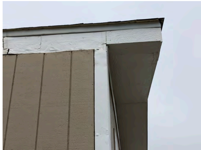
157 First Ave - No roof overhang. Typical of original construction method for older units. Evidence of fascia wear and indications of maintenance. No evidence of any modification of structural roof or wall elements.
