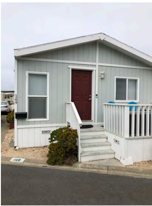
149 First Ave - Front elevation. Gable roof, no overhang, typical of original construction. T1-11 siding typical of original construction. No indication of modification to structural roof or wall elements.
