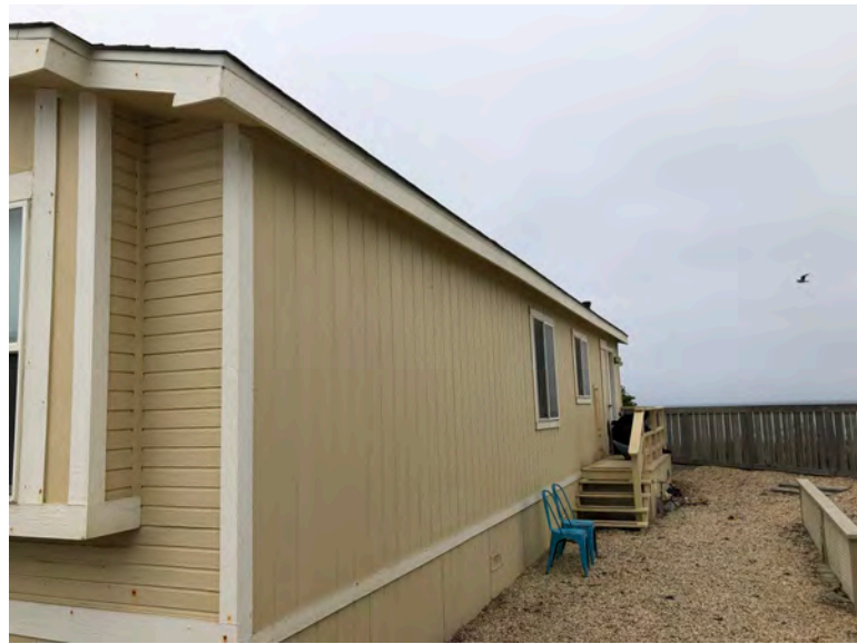
580 Fifth Ave - Side view. T1-11 siding typical of original construction. Evidence of non-structural repair and maintenance (e.g., caulking, sealing) of T1-11 wall covering. No indication that removal or replacement of structural wall framing has occurred.
