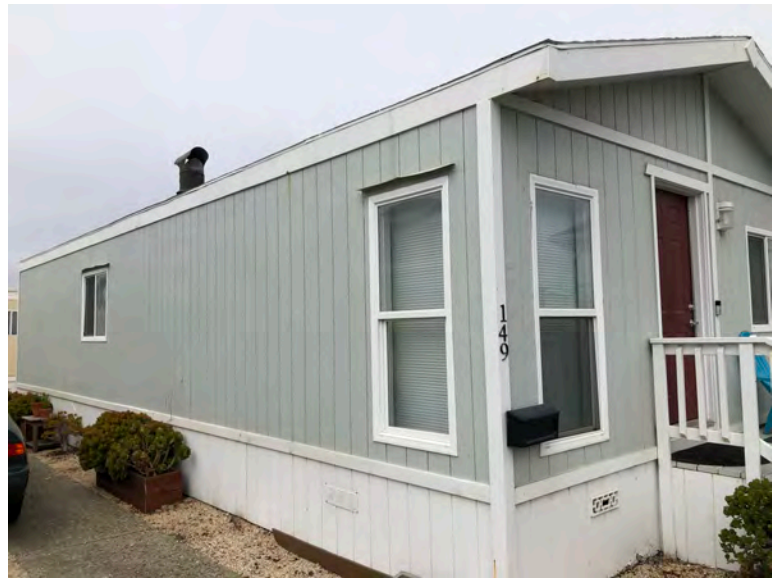
149 First Ave - Left side elevation. Gable roof, no overhang. Roof replacement likely would have included overhang. T1-11 siding typical of original construction. No indication that removal or replacement of structural wall framing has occurred.
