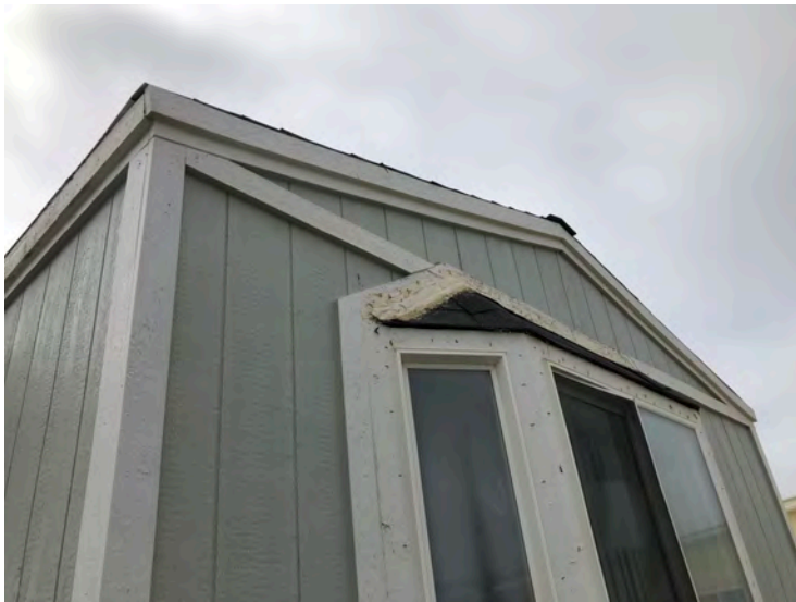
345 Third Ave - Gable roof, no overhang. T1-11 siding typical of original construction. Fascia detail at roof reflecting non-structural repair and maintenance, including re-painting. If roof structural framing had been replaced, boxed eave and fascia would not show similar wear. Replacement of roof elements likely would have included overhang.
