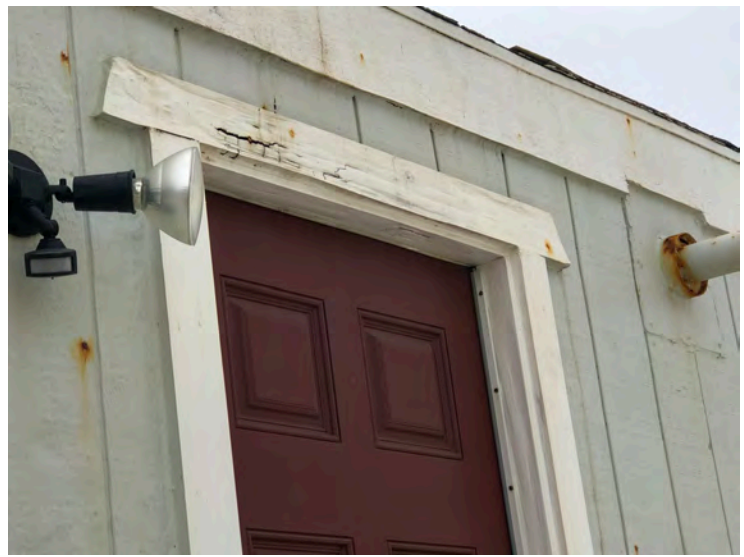
149 First Ave - Moulding over entry. Gable end roof with no overhang typical of original construction. Some wood rot over moulding. No evidence of modification to roof framing. If structural roof elements had been replaced, an overhang likely would have been included to further protect siding elements.
