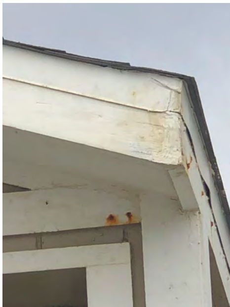
332 Third Ave - Fascia detail at roof. Fascia typical of original construction. Evidence of fascia wear and indications of maintenance, including caulking and re-painting. No evidence of any modifications to structural roof or wall elements. Roof replacement likely would have included overhang.
