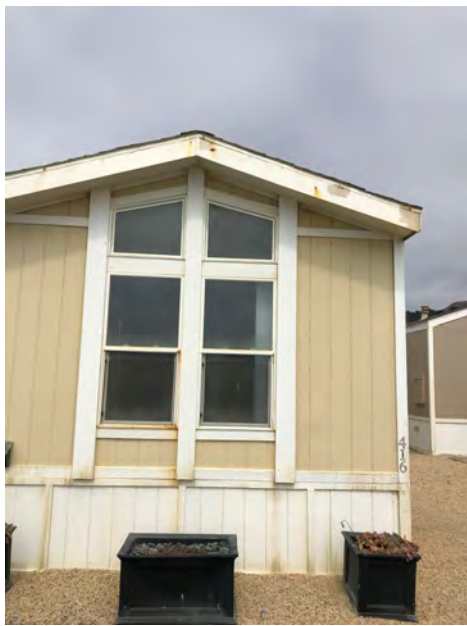
416 Fourth Ave - Front elevation. Materials and gable roof with little or no overhang typical of original construction. No indication that removal or replacement of structural roofing has occurred. Replacement would have had significant impact on wall framing and interiors and likely would have been built with an overhang.
