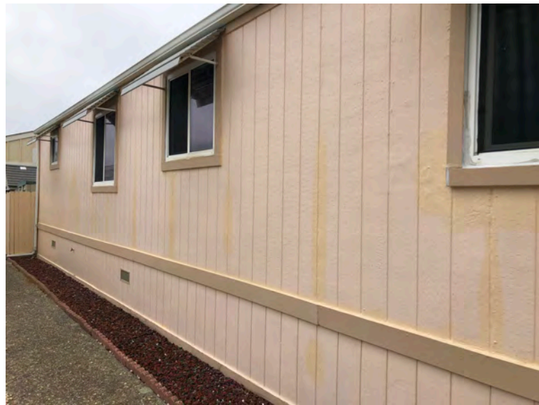
249 Second Ave - Evidence of non-structural repair and maintenance (e.g., caulking, sealing) of T1-11 wall covering. No indication that any removal or replacement of structural wall framing has occurred. If wall framing had been replaced, siding would not show similar wear.
