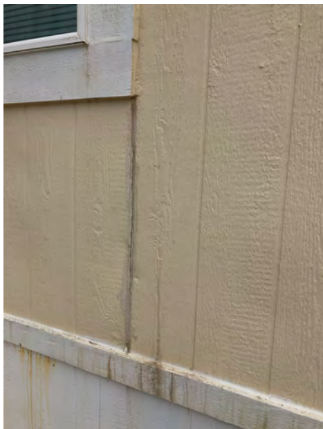
564 Fifth Ave - T1-11 siding typical of original construction. Evidence of non-structural repair and maintenance (e.g., caulking, sealing) of T1-11 wall covering. No indication that removal or replacement of structural wall framing has occurred.
