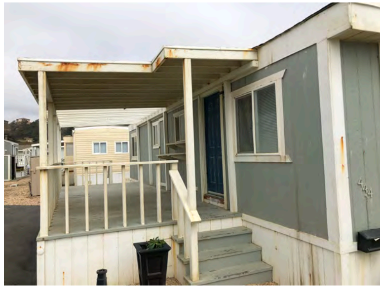
444 Fourth Ave - Side view, entry steps. T1-11 siding and fascia typical of original construction. Fascia wear at roof. If roof structural framing had been replaced, fascia would not show similar wear. Replacement of roof elements likely would have included overhang.
