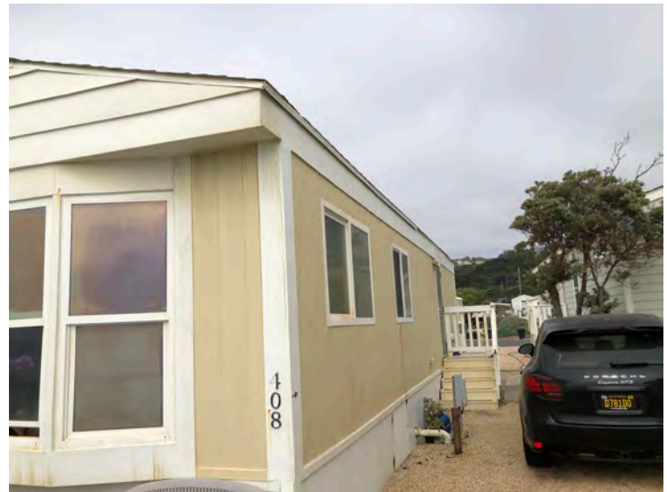
408 Fourth Ave - Side view, entry steps. Gable roof, no overhang. T1-11 siding typical of original construction. Evidence of patch and repair of existing T1-11 wall covering. No indication that removal or replacement of structural wall framing has occurred.
