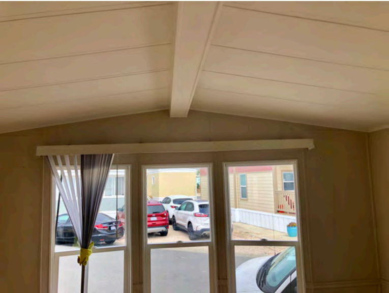
329 Third Ave - Interior elevation of open ceiling with boxed beam. Indicative of original gable construction. Interior finish of ceiling materials consistent with original construction.
