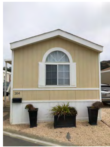
204 Second Ave - Front elevation with side entrance ("shotgun installation") Materials and gable roof with little or no overhang typical of original construction. No indication that any removal or replacement of structural roof framing has occurred. Replacement would have had significant impact on wall framing and interiors and likely would have been constructed with an overhang.
