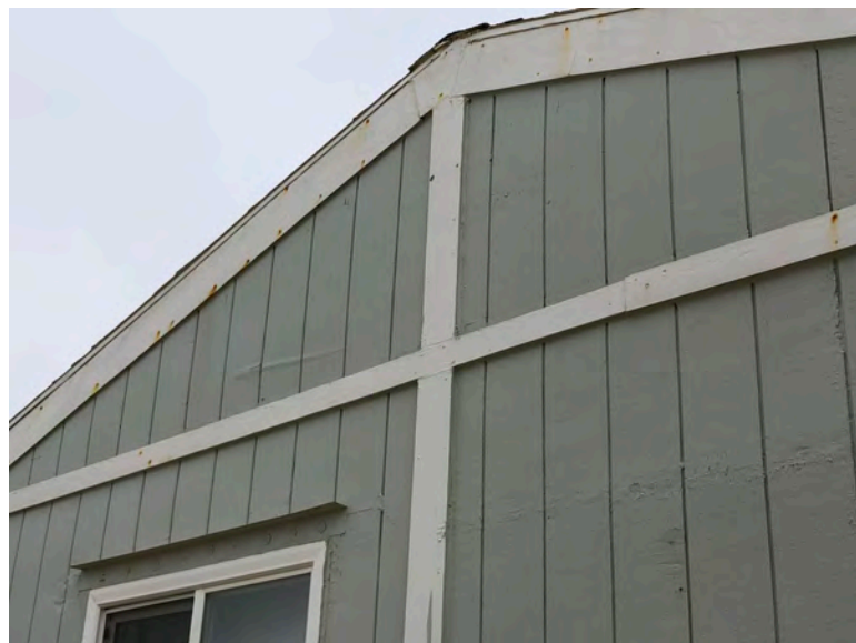
149 First Ave - Gable end of structure. Evidence of repair and maintenance of existing T1-11 wall covering without structural replacement. No evidence of any removal or replacement of structural roof framing system or wall elements.
