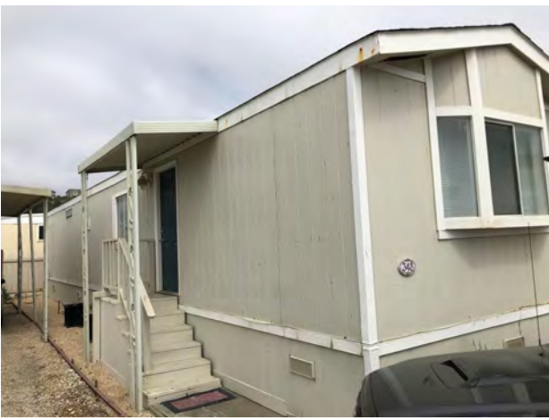
348 Third Ave - Side view, entry steps. Materials, pop out window, and gable roof with little or no overhang typical of original construction. No indication that removal or replacement of structural roof framing has occurred. Replacement would have had significant impact on wall framing and interiors and likely would have been constructed with an overhang.
