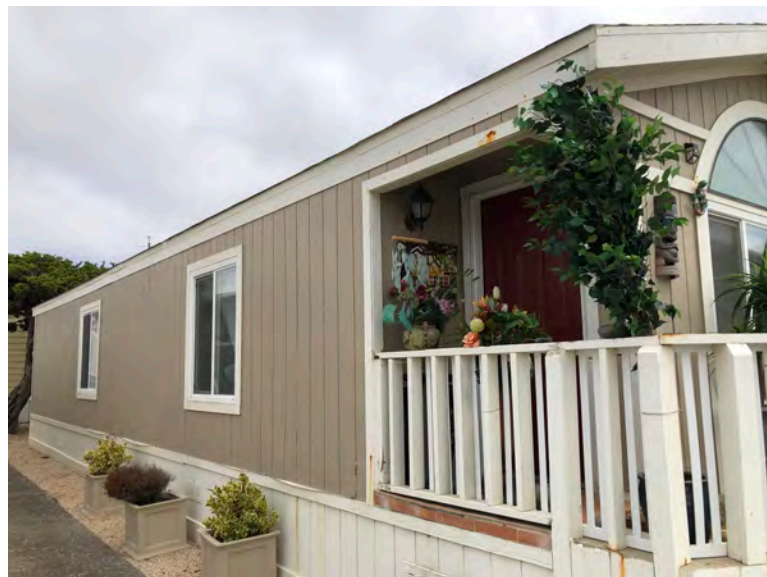
240 Second Ave - Side view with T1-11 siding. T1-11 siding typical of original construction. No indication that any removal or replacement of structural wall framing has occurred.
