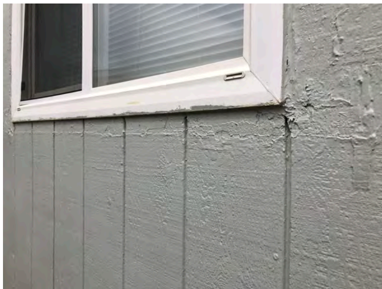
149 First Ave - Evidence of prior window replacement without modification of structural wall elements. Evidence of repair and maintenance to T1-11 wall surfacing without modification to existing structural wall framing elements. T1-11 wall covering typical of original construction.
