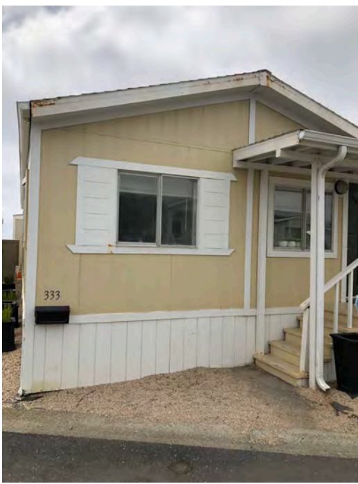
333 Third Ave - Front elevation. Gable roof with no overhang, typical of original construction. If roof framing had been replaced, likely would have been constructed with an overhang.
