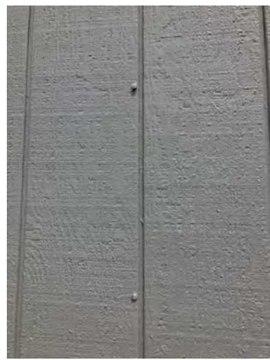
149 First Ave - Exterior. T1-11 siding wall covering. Evidence of maintenance of T1-11 covering. No indication that removal or replacement of structural wall framing has occurred. Modification of wall elements also would have had significant impact on roof framing.
