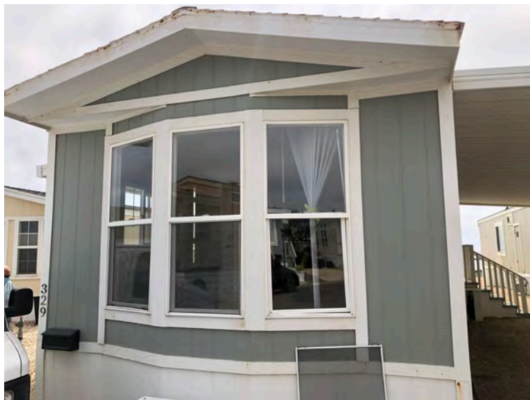
329 Third Ave - Front elevation. Gable roof construction with no overhang, typical of original construction. No indication that removal or replacement of structural roof framing has occurred. Replacement would have had significant impact on wall framing and interiors and likely would have been constructed with an overhang.
