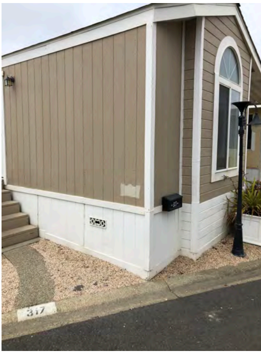
317 Third Ave - Front elevation. Gable roof with no overhang, typical of original construction. Roof replacement likely would have included overhang.
