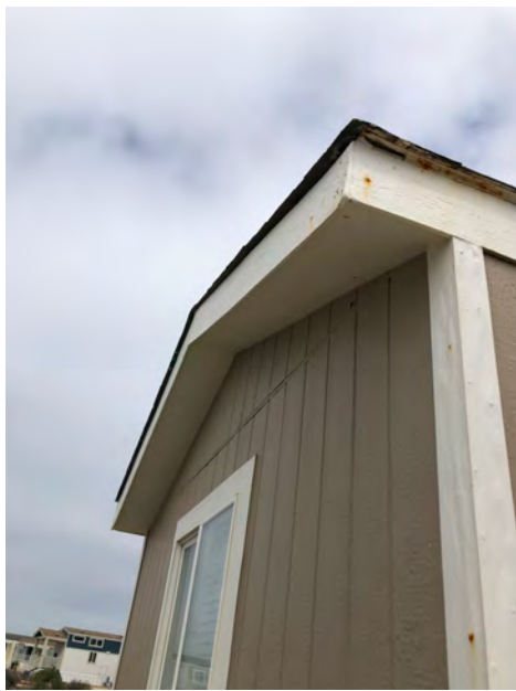
200 Second Ave - Fascia detail at roof. Fascia typical of original construction. If roof structural framing had been replaced, boxed eave and fascia would not show similar wear. Replacement of roof elements likely would have included overhang.
