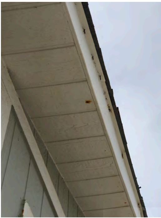
245 Second Ave - Boxed eaves at front elevation. Typical of older construction.
