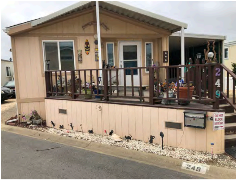
249 Second Ave - Front elevation. Gable roof construction with no overhang, typical of original construction. No indication that removal or replacement of structural roof framing has occurred. Replacement would have had significant impact on wall framing and interiors and likely would have been constructed with an overhang.
