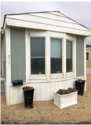
444 Fourth Ave - Front elevation with side entrance ("shotgun installation"). Gable roof with no overhang typical of original unit. No evidence of any modifications to structural roof elements. Roof replacement would have had significant impact on wall framing and interiors and likely would have included a roof overhang.
