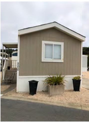
200 Second Ave - Front elevation with side entrance ("shotgun installation"). Materials and gable roof with little or no overhang typical of original construction. No indication that any removal or replacement of structural roof framing has occurred. Replacement would have had significant impact on wall framing and interiors and likely would have been constructed with an overhang.
