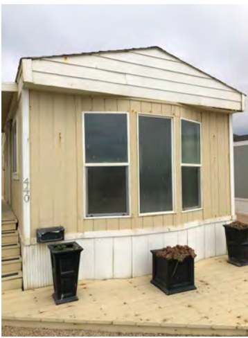
440 Fourth Ave - Front elevation with side entrance ("shotgun installation"). Gable roof with no overhang typical of original unit. No evidence of any modifications to structural roof elements. Roof replacement would have had significant impact on wall framing and interiors and likely would have included a roof overhang.
