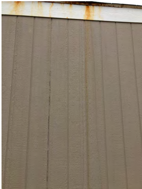
200 Second Ave - Existing T1-11 siding reflecting non-structural repair and maintenance.
