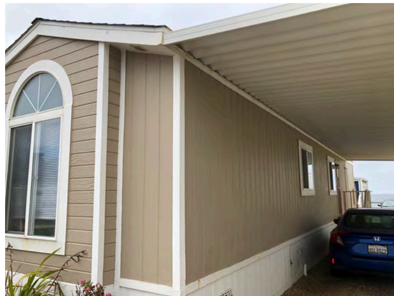
317 Third Ave - Side view with T1-11 siding. Evidence of non-structural repair and maintenance (e.g., caulking, sealing) of T1-11 wall covering. No indication that any removal or replacement of structural wall framing has occurred.
