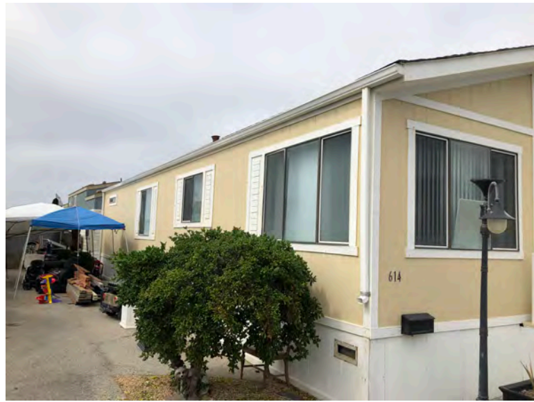
614 Sixth Ave - Side elevation. Materials and gable roof with little or no overhang typical of original construction. T1-11 siding typical of original construction. No indication that removal or replacement of structural roofing or wall elements has occurred. Replacement would have had significant impact on wall framing and interiors and likely would have been built with an overhang.
