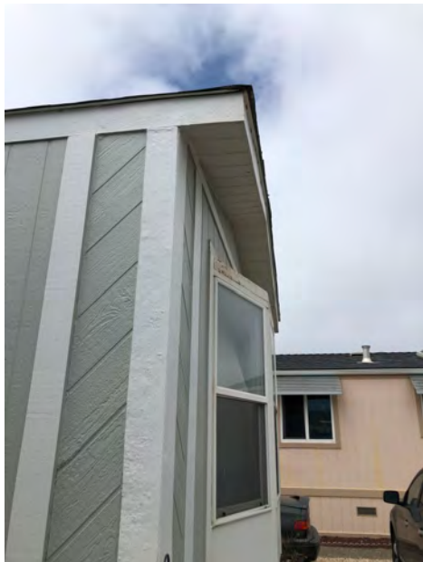
245 Second Ave - Fascia detail at roof reflecting non-structural repair and maintenance, including re-painting. Fascia typical of original construction. No evidence of any modifications to structural roof or wall elements. If roof structural framing had been replaced, boxed eave and fascia would not show similar wear. Replacement of roof elements likely would have included overhang.
