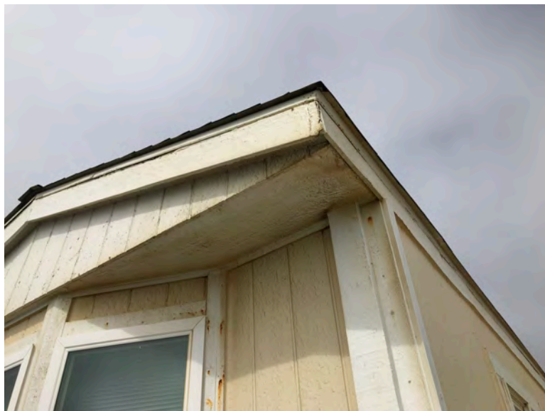
404 Fourth Ave - Gable roof, no overhang. T1-11 siding typical of original construction. Fascia detail at roof reflecting non-structural repair and maintenance. Fascia typical of original construction.
