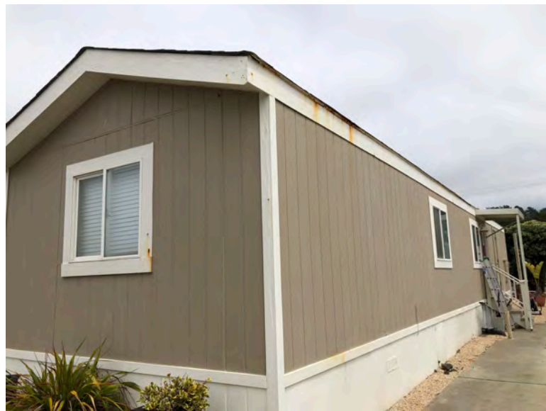
200 Second Ave - Side view with T1-11 siding. Evidence of repair and maintenance (e.g., caulking, sealing) of T1-11 wall-covering. No indication that removal or replacement of structural wall framing has occurred.
