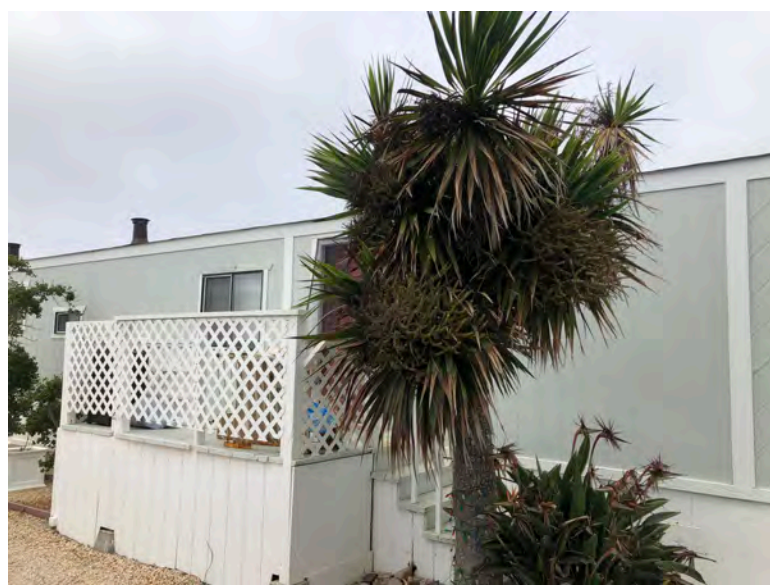
245 Second Ave - Side view with T1-11 siding. Evidence of non-structural repair and maintenance (e.g. caulking, sealing) of T1-11 wall covering. T1-11 siding typical of original construction. No indication that any removal or replacement of structural wall framing has occurred.
