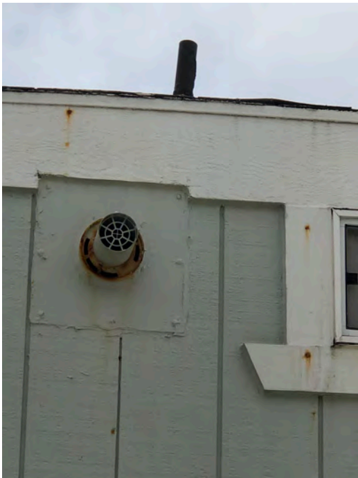
149 First Ave - Original heater vent installed in existing wall, indicative of original construction.
