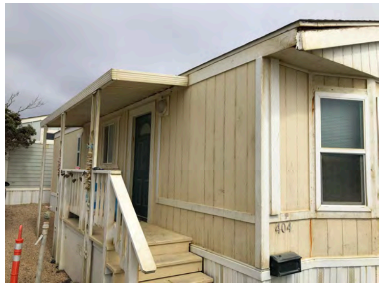
404 Fourth Ave - Side view, entry steps. Materials and gable roof with little or no overhang typical of original construction. No indication that removal or replacement of structural roofing has occurred. Replacement would have had significant impact on wall framing and interiors and likely would have been built with an overhang.
