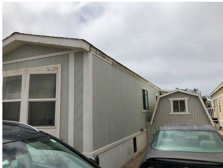
245 Second Ave - Side View with T1-11 siding. Evidence of non-structural repair and maintenance (e.g. caulking, sealing) of T1-11 covering. No indication that any removal or replacement of structural wall framing has occurred.
