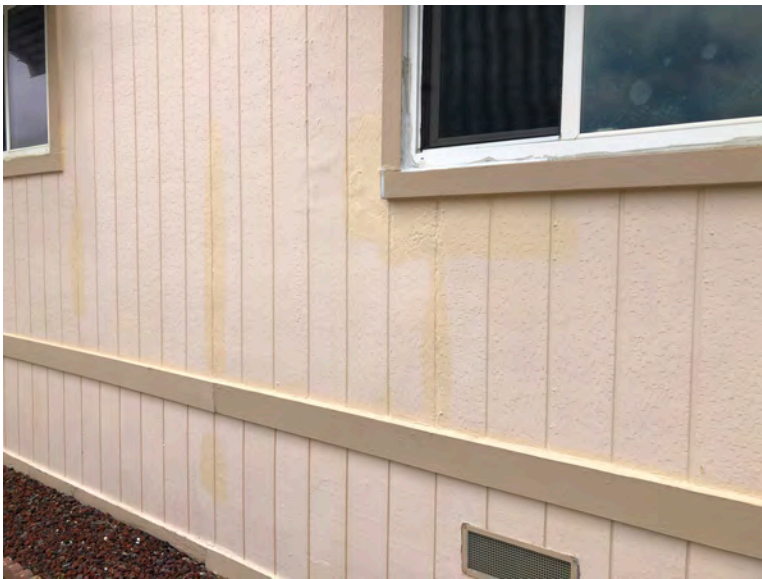
249 Second Ave - Evidence of non-structural repair and maintenance (e.g., caulking, sealing) of T1-11 wall covering. T1-11 siding typical of original construction. No indication that any removal or replacement of structural wall framing has occurred. If wall framing had been replaced, siding would not show similar wear.
