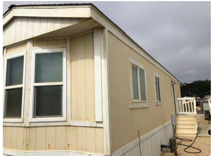
404 Fourth Ave - Side view, entry steps. Gable roof, no overhang. T1-11 siding typical of original construction. Evidence of patch and repair work of existing T1-11 wall covering. No indication that removal or replacement of structural wall framing has occurred.
