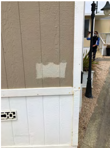
317 Third Ave - Side view with T1-11 siding. Evidence of non-structural repair and maintenance (e.g., caulking, sealing) of T1-11 wall covering. No indication that any removal or replacement of structural wall framing has occurred. Note old style wall vent, typical of original construction.
