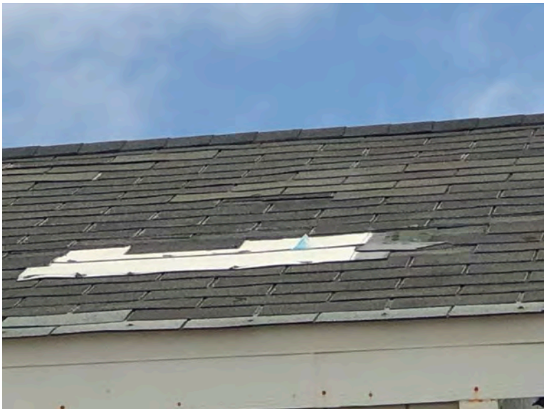
245 Second Ave - Missing shingles at roof. Evidence of some shingle replacement. Typical non-structural repair and maintenance item due to location on roof of unit and weathering.
