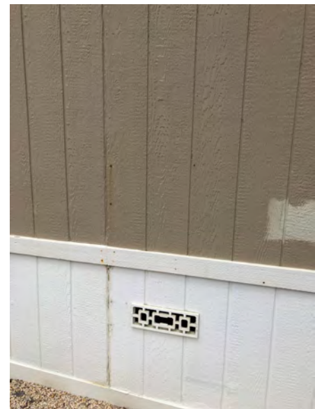
317 Third Ave - Side view with T1-11 siding. Evidence of non-structural repair and maintenance (e.g., caulking, sealing) of T1-11 wall covering. No indication that any removal or replacement of structural wall framing has occurred. Note old style wall vent, typical of original construction.
