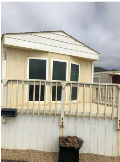
432 Fourth Ave - Materials and gable roof with little or no overhang typical of original construction. No indication that removal or replacement of structural roofing has occurred. Replacement would have had significant impact on framing and likely would have been built with an overhang.
