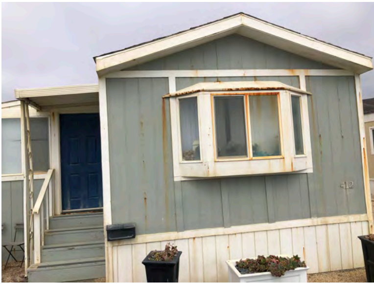
412 Fourth Ave - Front elevation. Gable roof with no overhang, pop out window, typical of original construction. If roof framing had been replaced, likely would have been built with an overhang.
