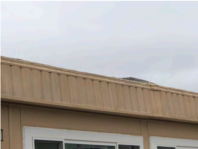
622 Sixth Ave - Original metal wall covering at roof parapet.
