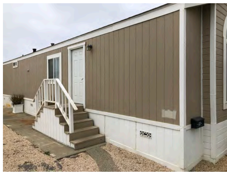
317 Third Ave - Side view with T1-11 siding. Evidence of non-structural repair and maintenance (e.g., caulking, sealing) of T1-11 wall covering. T1-11 siding typical of original construction. No indication that removal or replacement of structural wall framing has occurred.
