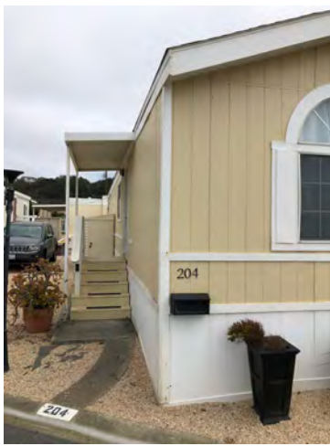
204 Second Ave - Front elevation with side entrance ("shotgun installation"). Materials and gable roof with little or no overhang typical of original construction. No indication that removal or replacement of structural roof framing has occurred. Replacement would have had significant impact on wall framing and interiors and likely would have been constructed with an overhang.
