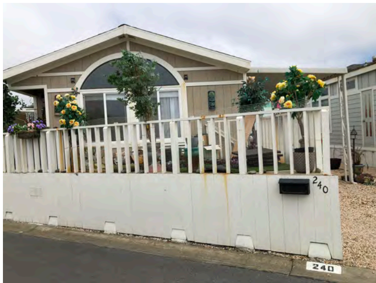
240 Second Ave - Front view. Materials and gable roof with little or no overhang typical of original construction. No indication that removal or replacement of structural roof framing has occurred. Replacement would have had significant impact on wall framing and interiors and likely would have been constructed with an overhang.
