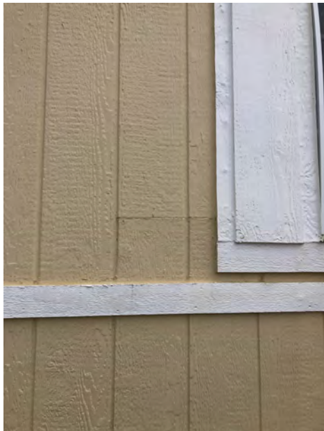
204 Second Ave - 200 Second Ave - Evidence of non-structural repair and maintenance (e.g., caulking, sealing) of T1-11 wall covering. T1-11 siding typical of original construction. No indication that any removal or replacement of structural wall framing has occurred.
