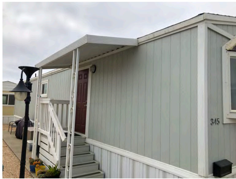
345 Third Ave - Side view, entry steps. Gable roof, no overhang. T1-11 siding typical of original construction. No indication that removal or replacement of structural wall framing has occurred.
