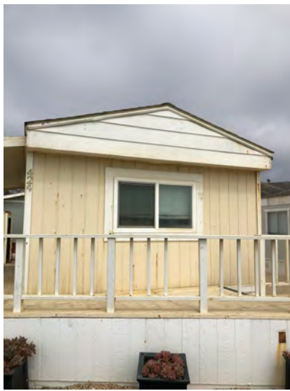
424 Fourth Ave - Front elevation with side entrance ("shotgun installation"). Gable roof with no overhang typical of original unit. No evidence of any modifications to structural roof elements. Roof replacement would have had significant impact on wall framing and interiors and likely would have included a roof overhang.
