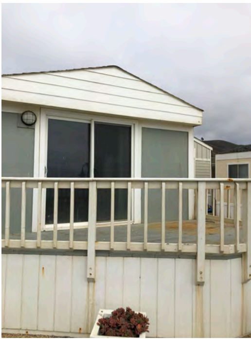
436 Fourth Ave - Front elevation. Gable roof with no overhang, pop out window, typical of original construction. If roof framing had been replaced, likely would have been built with an overhang.
