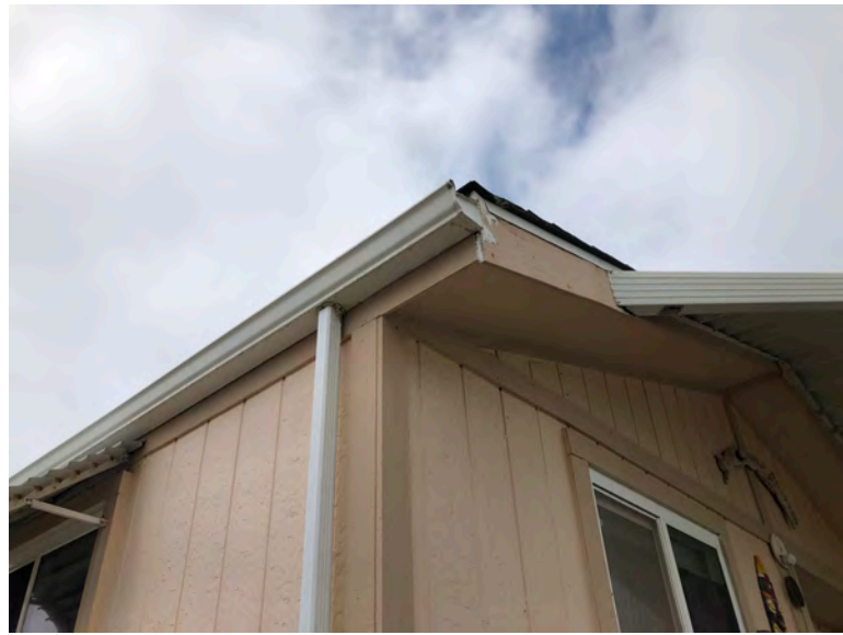
249 Second Ave - Fascia detail at roof. Fascia typical of original construction. Evidence of fascia wear and indications of maintenance, including re-painting. No evidence of any modifications to structural roof or wall elements. If roof structural framing had been replaced, boxed eave and fascia would not show similar wear.
