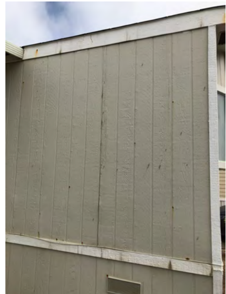
348 Third Ave - Exterior T1-11 siding wall covering. Evidence of non-structural repair and maintenance (e.g., caulking, sealing) of T1-11 wall covering. T1-11 siding typical of original construction. No indication that removal or replacement of structural wall framing has occurred.
