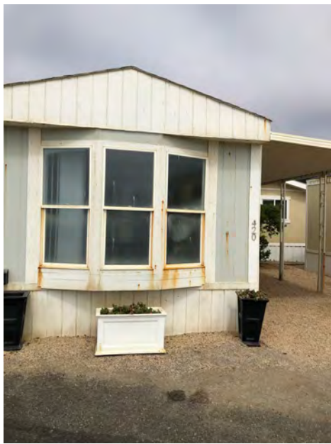
420 Fourth Ave - Materials, pop out window, and gable roof with little or no overhang typical of original construction. No indication that removal or replacement of structural roofing has occurred. Replacement would have had significant impact on wall framing and interiors and likely would have been built with an overhang.
