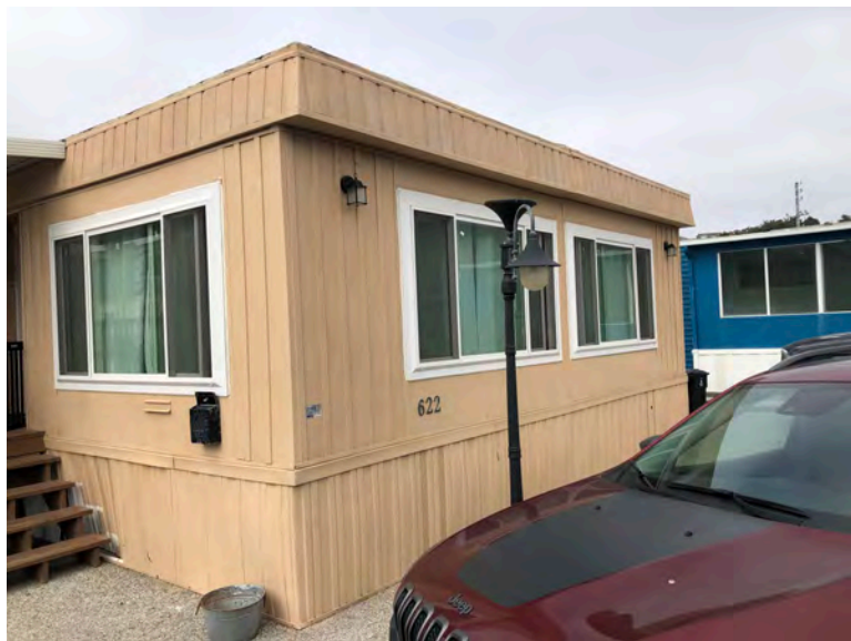
622 Sixth Ave - Mansard roof with flat roof at center. Original framing materials at walls and parapet indicating original construction. No indication that removal or replacement of structural roof or wall framing elements has occurred.
