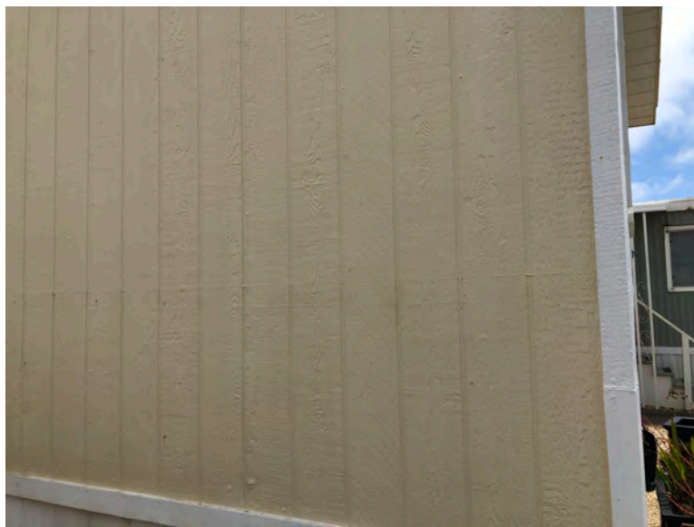
220 Second Ave - Evidence of non-structural repair and maintenance (e.g., caulking, sealing) of T1-11 wall covering. No indication that any removal or replacement of structural wall framing has occurred.
