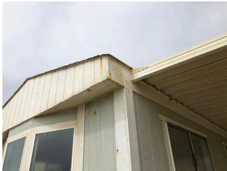
420 Fourth Ave - Gable roof, no overhang. T1-11 siding typical of original construction. Fascia wear at roof. If roof structural framing had been replaced, fascia would not show similar wear. Replacement of roof elements likely would have included overhang.
