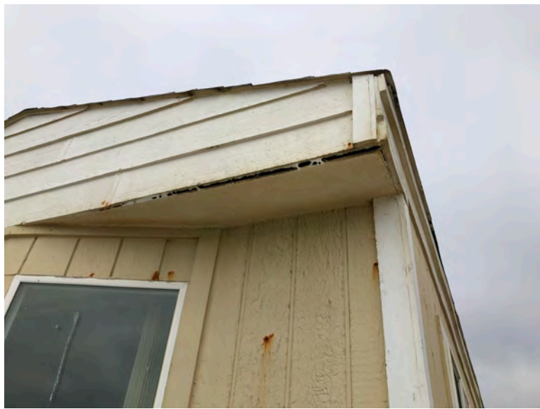
440 Fourth Ave - Gable roof, no overhang. T1-11 siding typical of original construction. Fascia detail at roof reflecting repair and maintenance. If roof structural framing had been replaced, fascia would not show similar wear. Replacement of roof elements likely would have included overhang.
