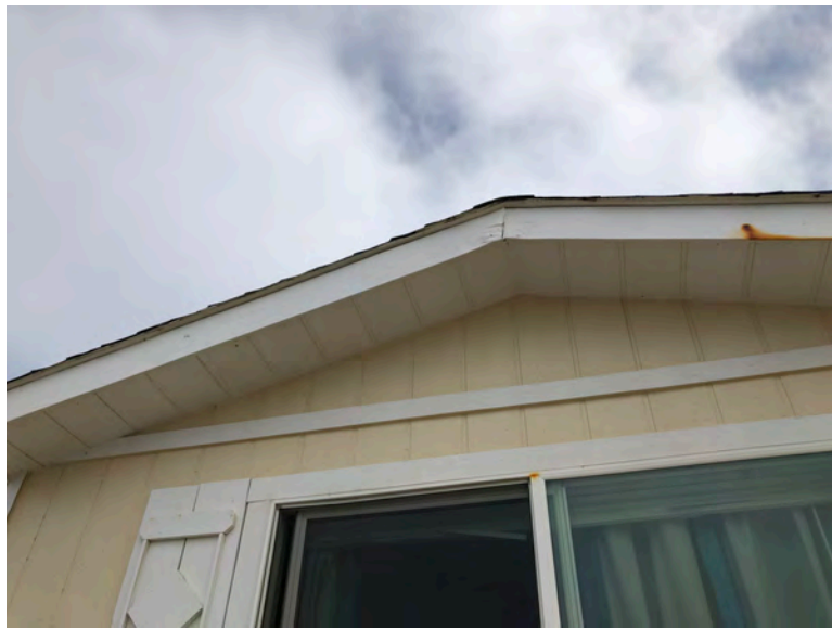
220 Second Ave - Fascia detail at roof. Fascia typical of original construction. Evidence of fascia wear and indications of maintenance, including re-painting. No evidence of any modifications to structural roof or wall elements. If roof structural framing had been replaced, boxed eave and fascia would not show similar wear. Replacement of roof elements likely would have included overhang.
