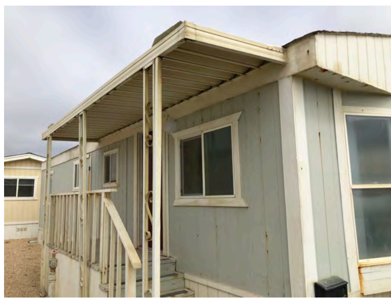
420 Fourth Ave - Side elevation. T1-11 siding typical of original construction. Evidence of repair and maintenance of T1-11 wall covering. Fascia wear at roof. If roof structural framing had been replaced, fascia would not show similar wear. Replacement of roof elements likely would have included overhang. Evidence of prior window replacement without modification to structural elements.
