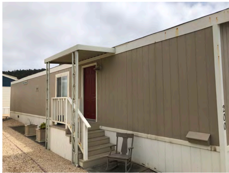
200 Second Ave - Side view with T1-11 siding. T1-11 siding typical of original construction. Evidence of repair and maintenance (e.g., caulking, sealing) of T1-11 wall covering. No indication that any removal or replacement of structural wall framing has occurred.
