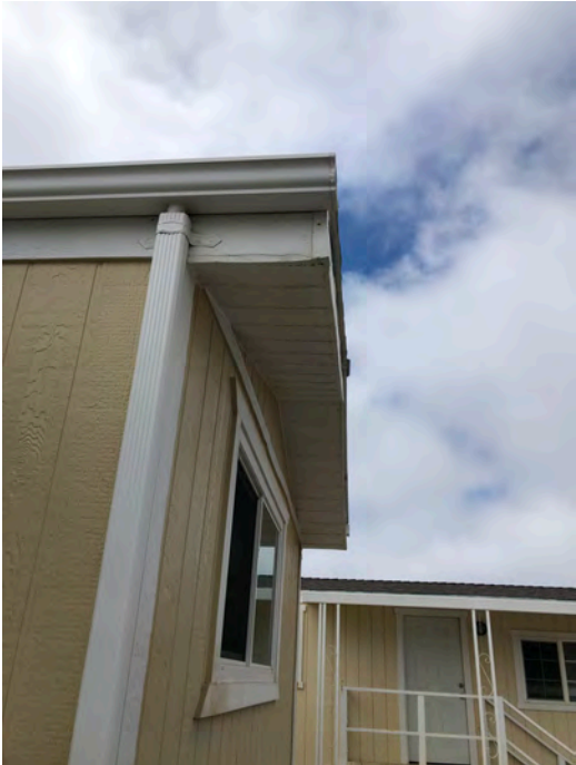
321 Third Ave - Fascia detail at roof with boxed eave. No roof overhang, typical of original construction. No indication of changes to structural roof framing.
