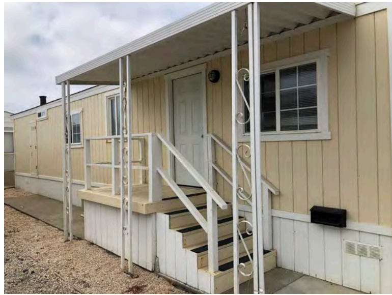
325 Third Ave - Entrance at side elevation. No roof overhang, typical of original construction. No indication that any removal or replacement of structural roof framing has occurred. Replacement would have had significant impact on wall framing and interiors.
