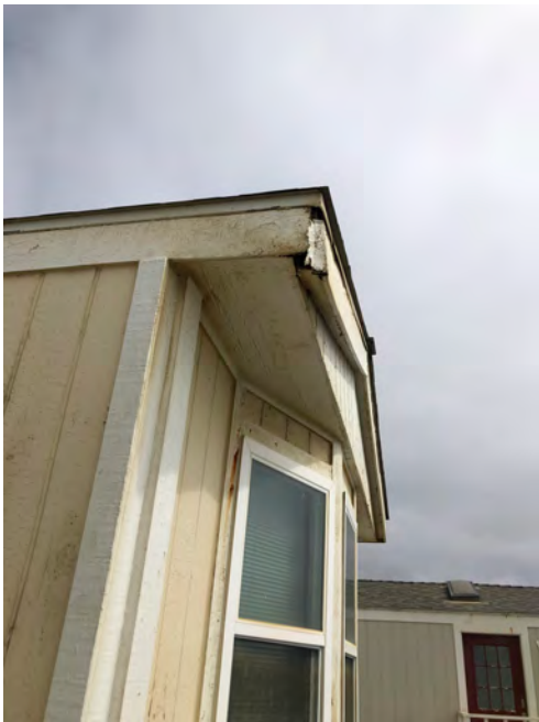
404 Fourth Ave - Gable roof, no overhang. T1-11 siding typical of original construction. Fascia typical of original construction. Fascia wear at roof and indications of repair and maintenance. If roof structural framing had been replaced, boxed eave and fascia would not show similar wear. Replacement of roof elements likely would have included overhang.
