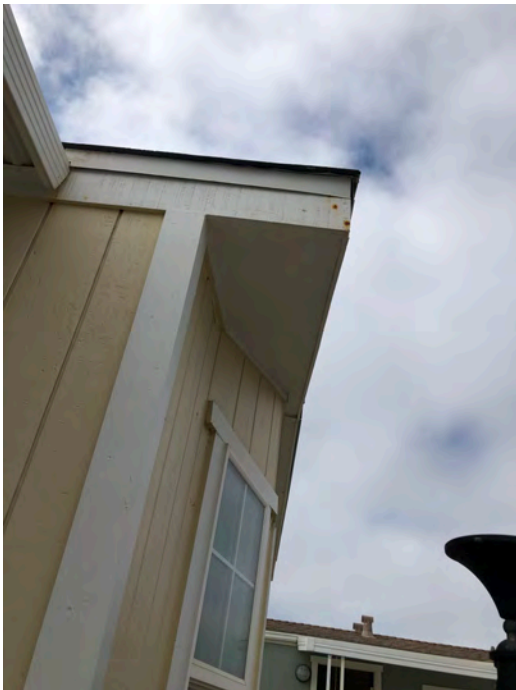
325 Third Ave - Boxed soffit at front gable, no roof overhang at side, typical of original construction.
