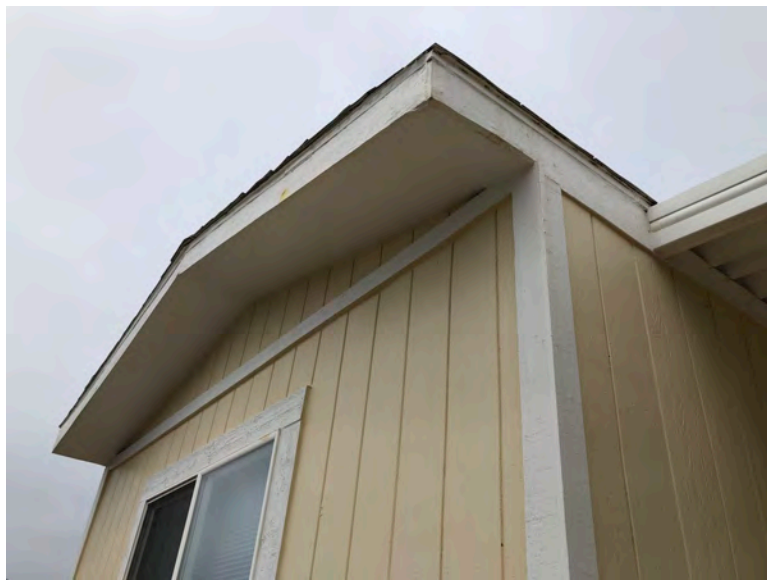
564 Fifth Ave - Side view of front elevation, gable roof construction with no eaves at side and boxed eave at front. Typical of older model original construction
