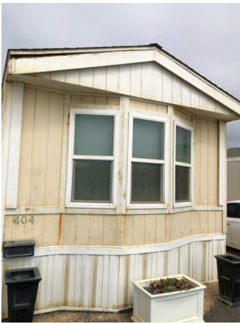
404 Fourth Ave - Front elevation. Gable roof with no overhang, pop out window, typical of original construction. If roof framing had been replaced, likely would have been built with an overhang.
