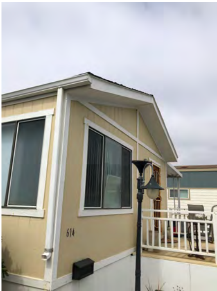
614 Sixth Ave - Gable roof with no overhang. Gable roof construction with no eaves at side and boxed eave at front. Typical of older model original construction. No indication that removal or replacement of structural roofing has occurred.
