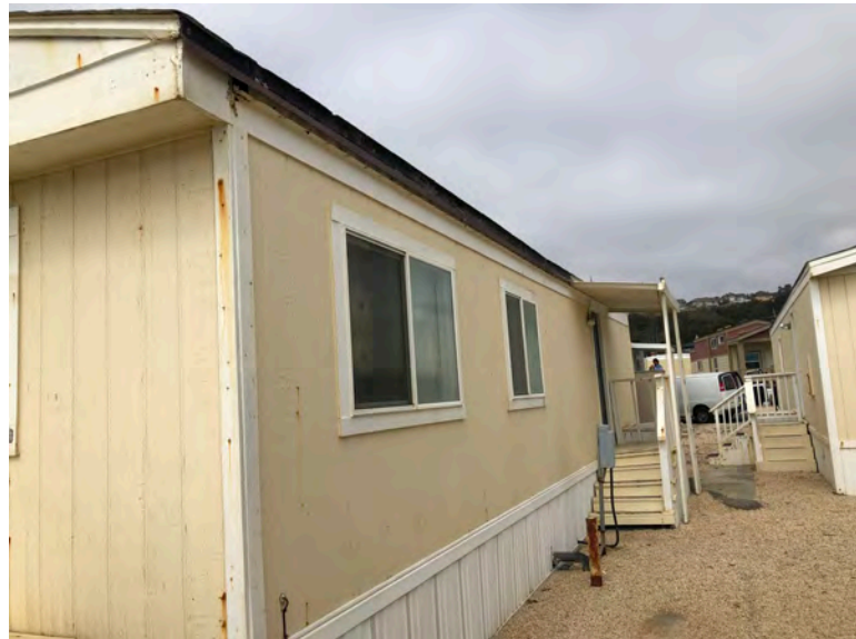
424 Fourth Ave - Side elevation, entry steps. Gable roof, no overhang. T1-11 siding typical of original construction. No indication that any removal or replacement of structural wall framing has occurred.
