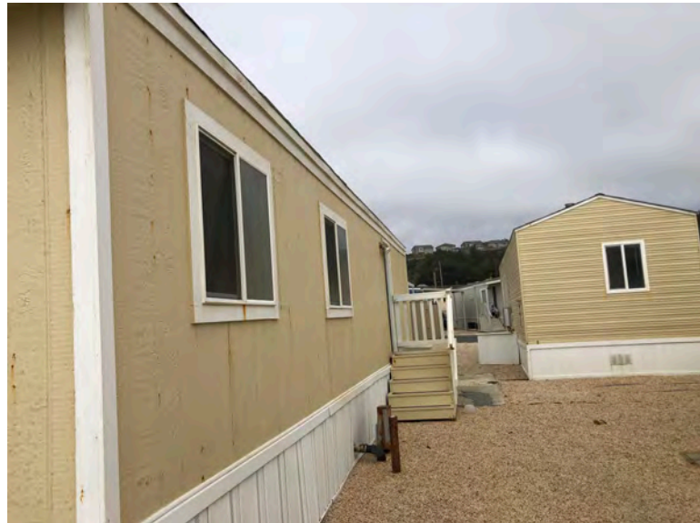
440 Fourth Ave - Side elevation. T1-11 siding typical of original construction. Evidence of patch and repair of wall surface without modification of structural elements. Fascia wear at roof. If roof structural framing had been replaced, fascia would not show similar wear. Replacement of roof elements likely would have included overhang.
