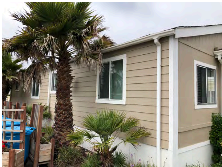
229 Second Ave - Side view with lapped siding. No indication that removal or replacement of structural wall framing or siding elements has occurred.
