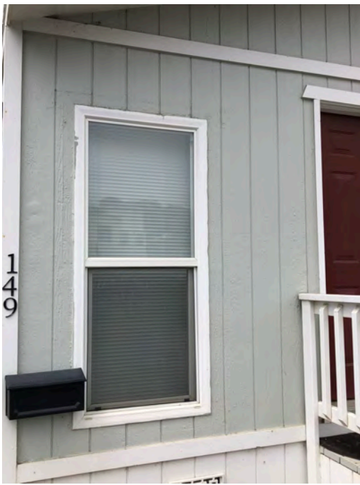
149 First Ave - Front elevation. Evidence of prior window replacement without modification of structural wall elements.
