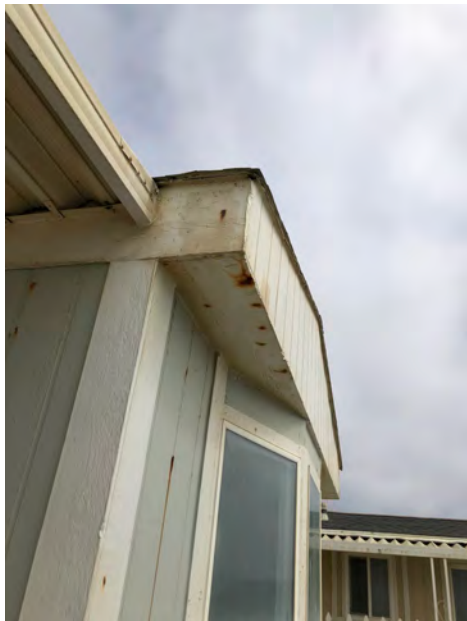
420 Fourth Ave - Gable roof, no overhang. T1-11 siding and fascia typical of original construction. Fascia wear at roof and indications of repair and maintenance. If roof structural framing had been replaced, fascia would not show similar wear. Replacement of roof elements likely would have included overhang.
