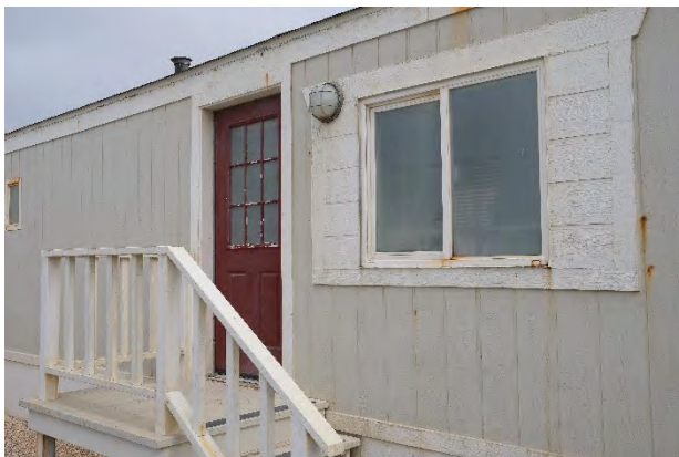
400 Fourth Ave - Gable roof, no overhang. T1-11 siding typical of original construction. Fascia typical of original construction. Fascia wear at roof. If roof structural framing had been replaced, boxed eave and fascia would not show similar wear. Replacement of roof elements likely would have included overhang.
