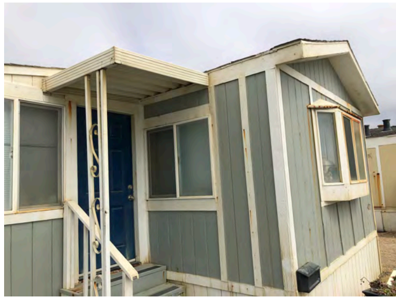
412 Fourth Ave - Materials and gable roof with little or no overhang typical of original construction. No indication that removal or replacement of structural roofing has occurred. Replacement would have had significant impact on wall framing and interiors and likely would have been built with an overhang.
