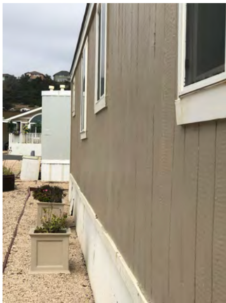
332 Third Ave - Side elevation. T1-11 siding material typical of original construction.
