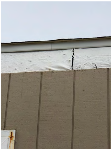
157 First Ave - Fascia typical of original construction. Evidence of fascia wear and indications of maintenance, including caulking and re-painting. No evidence of any modifications to structural roof or wall elements. Roof replacement likely would have included overhang.
