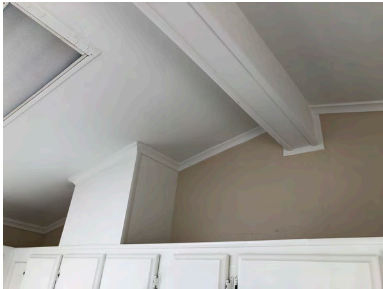
157 First Ave - Interior elevation of vaulted ceiling (from gable construction) over kitchen. No evidence of any structural modifications. Cabinets and trim are integral to the original construction.
