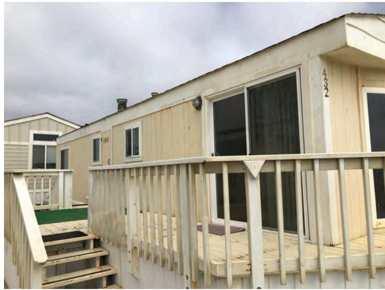
432 Fourth Ave - Side view. Materials and gable roof with little or no overhang typical of original construction. No indication that removal or replacement of structural roofing has occurred. Replacement would have had significant impact on wall framing and interiors and likely would have been built with an overhang.
