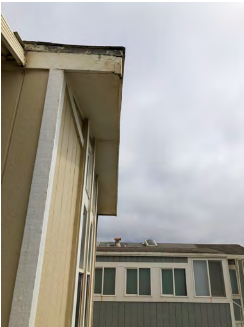
416 Fourth Ave - Gable roof, no overhang. T1-11 siding typical of original construction. Fascia wear at roof and indications of repair and maintenance. If roof structural framing had been replaced, fascia would not show similar wear. Replacement of roof elements likely would have included overhang.
