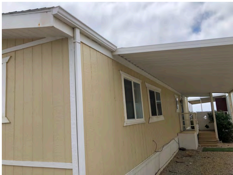
321 Third Ave - Side view with T1-11 siding. Evidence of non-structural repair and maintenance (e.g., caulking, sealing) of T1-11 wall covering. T1-11 siding typical of original construction. No indication that any removal or replacement of structural wall framing has occurred.
