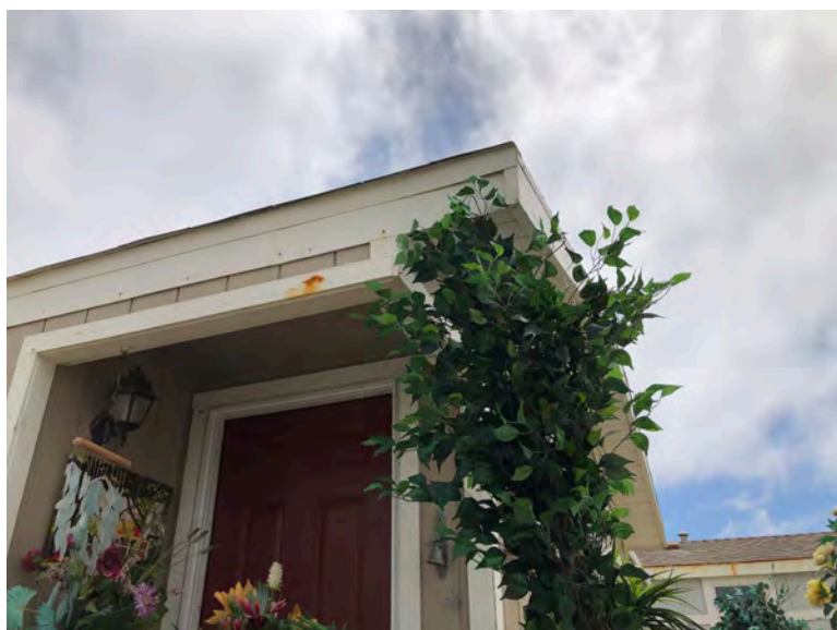
240 Second Ave - Side view of roof over front porch area, typical of original construction. No roof overhang.
