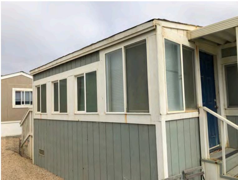
412 Fourth Ave - Gable roof, no overhang. T1-11 siding and fascia typical of original construction. Fascia wear at roof and indications of maintenance. No evidence of any modifications to structural roof or wall elements. If roof structural framing had been replaced, fascia would not show similar wear. Replacement of roof elements likely would have included overhang.
