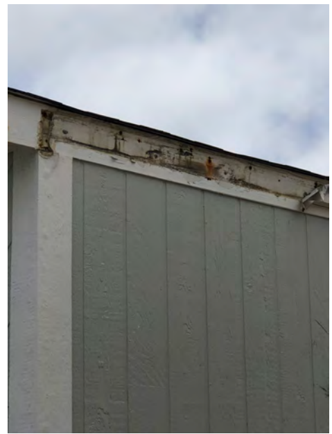
245 Second Ave - Fascia detail at roof. Fascia typical of original construction. Fascia shows wear s and reflects repair and maintenance, including re-painting. If roof structural framing had been replaced, boxed eave and fascia would not show similar wear. Replacement of roof elements likely would have included overhang.
