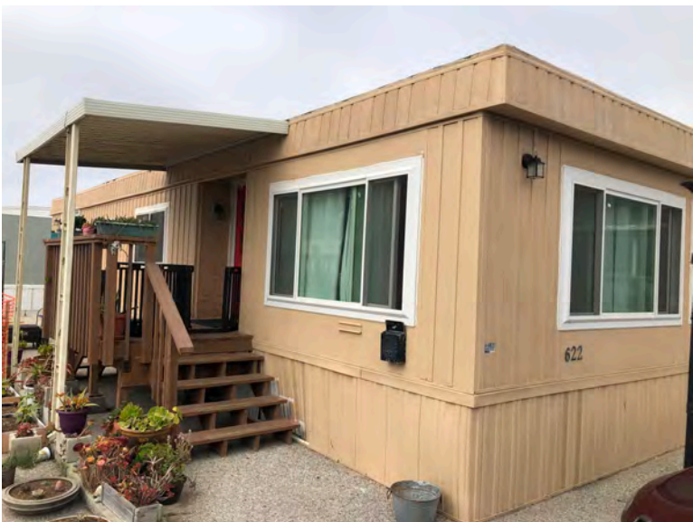
622 Sixth Ave - Side view with mansard roof (flat section in center), entry stairs. Original metal siding.
