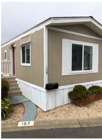
157 First Ave - Front Elevation with side entrance ("shotgun installation"). Gable roof with no overhang typical of original unit. No evidence of any modifications to structural roof elements. Roof replacement would have had significant impact on wall framing and interiors and likely would have included a roof overhang.
