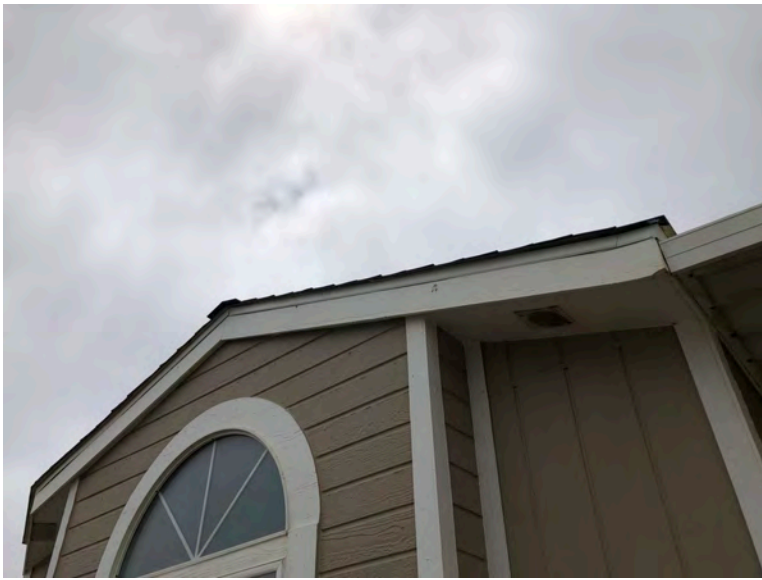
317 Third Ave - Fascia detail at roof with boxed eave, no overhang. Fascia typical of original construction. Note old style vent at boxed eave, typical of original construction.
