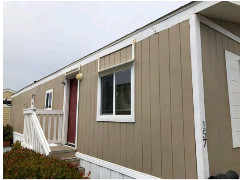
157 First Ave - Entry stairs. Evidence of prior window replacement without modification of structural wall elements. Gable roof with no overhang. T1-11 wall covering typical of original construction.
