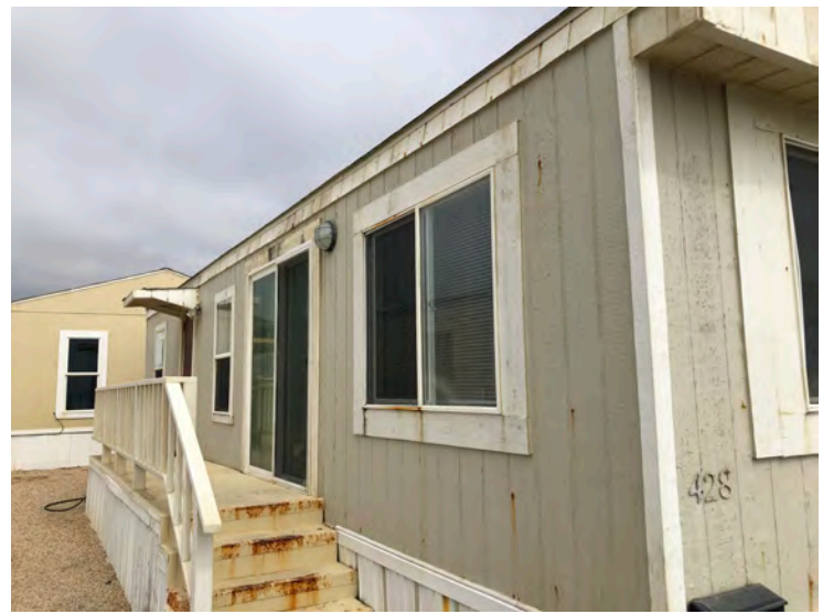
428 Fourth Ave - Side entrance. Materials and gable roof with little or no overhang typical of original construction. No indication that removal or replacement of structural roofing has occurred. Replacement would have had significant impact on wall framing and interiors and likely would have been built with an overhang.
