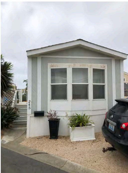
245 Second Ave - Front view. Gable roof with no overhang, typical of original construction. Roof replacement likely would have included overhang. Pop out window.
