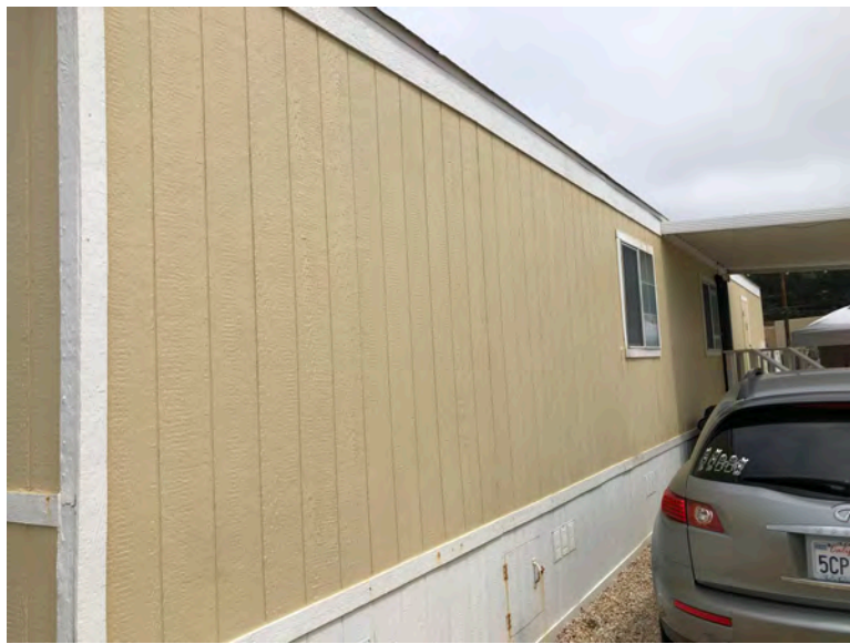
204 Second Ave - Side view with T1-11 siding. Evidence of non-structural repair and maintenance (e.g., caulking, sealing) of T1-11 wall covering. T1-11 siding typical of original construction. No indication that any removal or replacement of structural wall framing has occurred.
