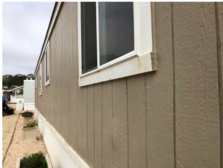
332 Third Ave - Side elevation. T1-11 siding material typical of original construction.
