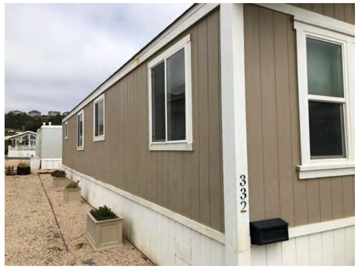
332 Third Ave - Side view with T1-11 siding. Evidence of non-structural repair and maintenance (e.g., caulking, sealing) of T1-11 wall covering. T1-11 siding typical of original construction. No indication that removal or replacement of structural wall framing has occurred.
