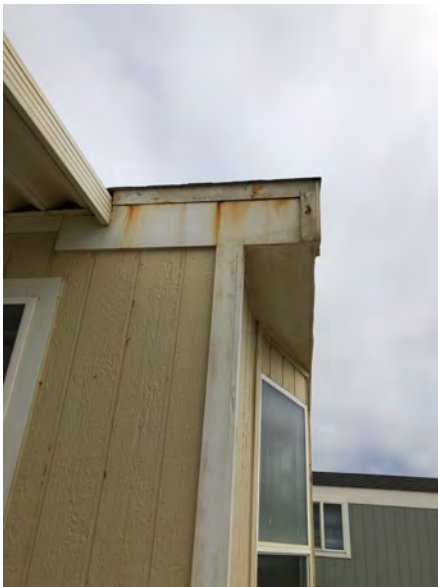
440 Fourth Ave - Gable roof, no overhang. T1-11 siding typical of original construction. Fascia wear at roof. If roof structural framing had been replaced, fascia would not show similar wear. Replacement of roof elements likely would have included overhang.
