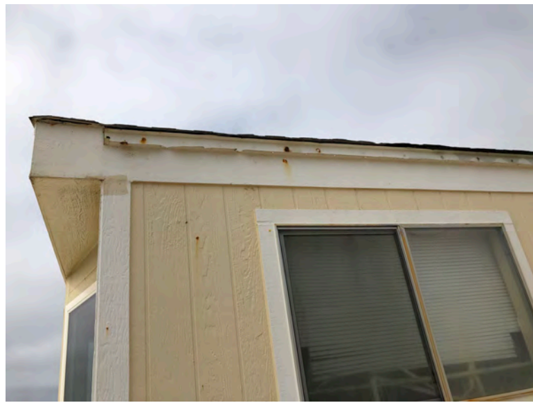
432 Fourth Ave - Side elevation. Gable roof, no overhang. T1-11 siding typical of original construction. No indication that removal or replacement of structural wall framing has occurred.
