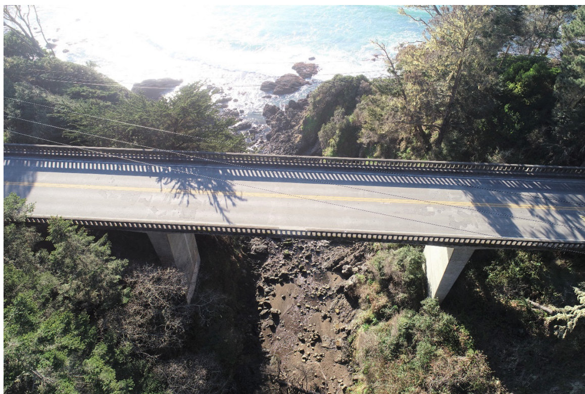
Figure 4: View of the existing Jack Peters Creek Bridge and piers anchored into bedrock (Source: Caltrans).
