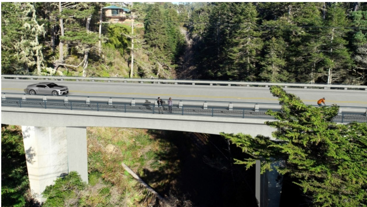
Figure 7: View of Proposed Bridge with bike shoulders, pedestrian path, and strengthened piers (Source: Caltrans).
