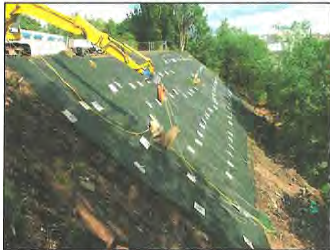
Soil Nail Stabilization of Slope
