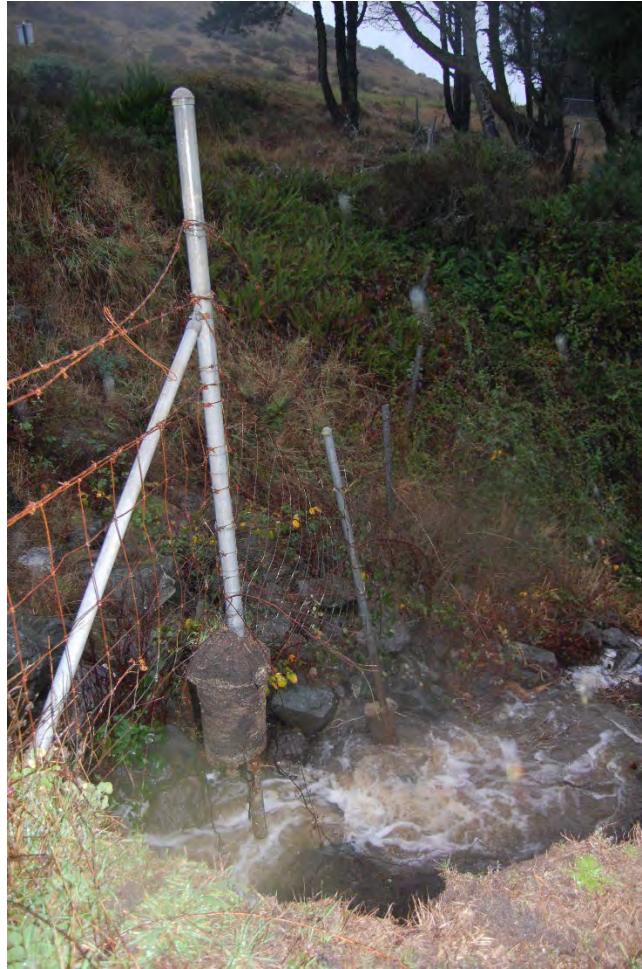
Looking towards southern side back in 2008, also showing erosion, rock migration and steepening of the slope.
