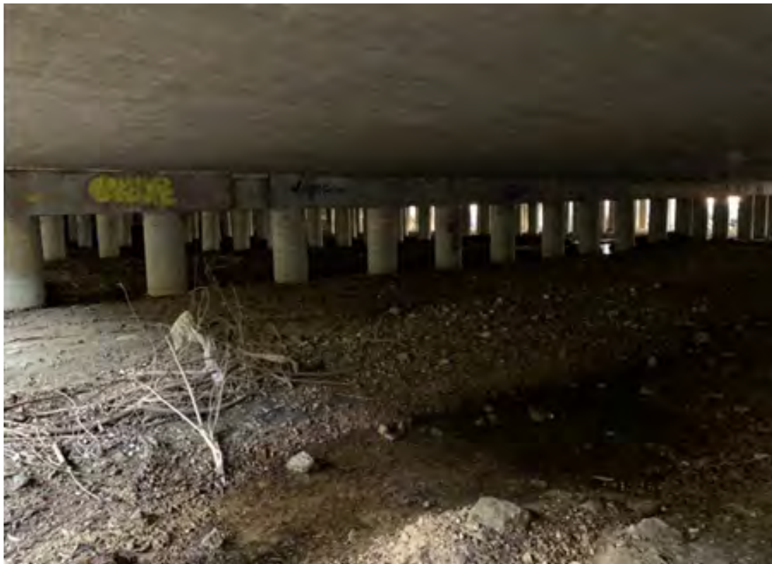
Looking under Interstate 5. Source: Caltrans.
