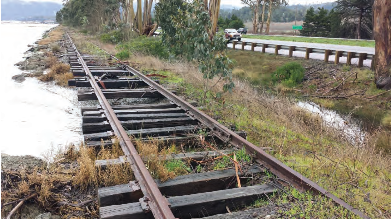
Photo 17 (February 9, 2017): View facing northeast of erosion of railroad prism (Segment 7).
