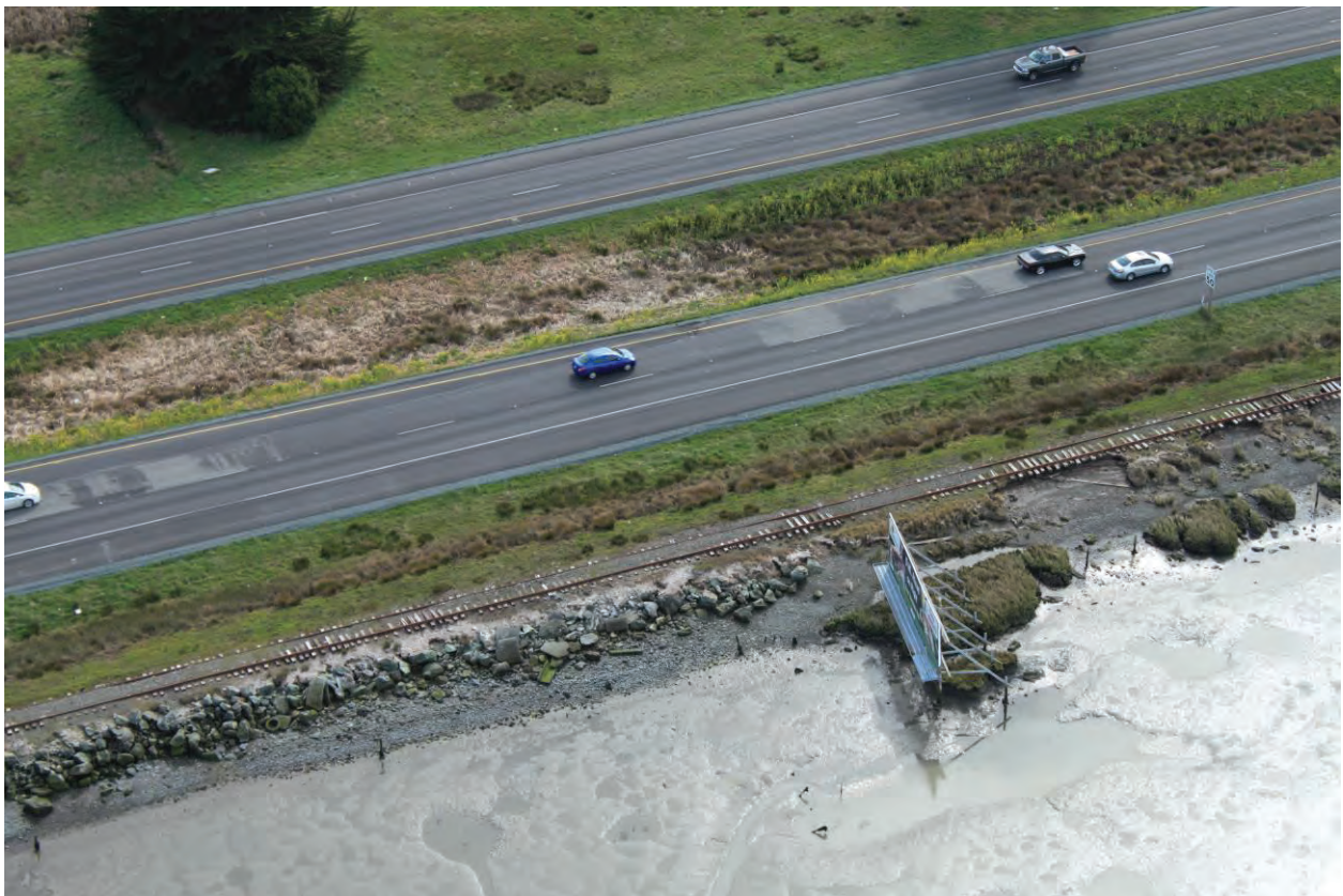
Photo 30 (February 25, 2014): View facing east of erosion of shoreline and railroad prism (Segment 8).
