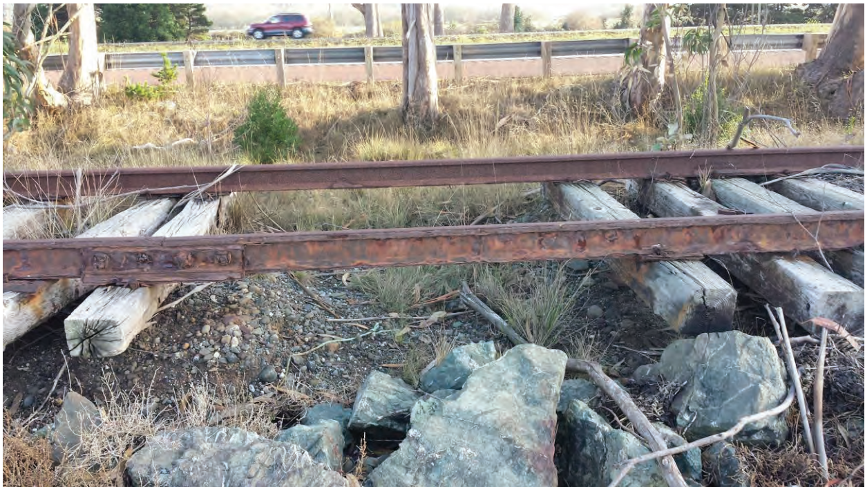
Photo 20 (December 1, 2017): View facing east of erosion of railroad prism (Segment 7).
