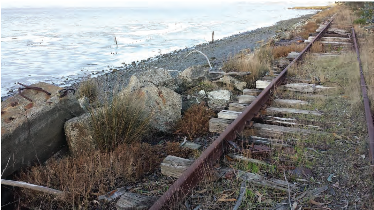
Photo 18 (December 1, 2017): View facing north of disarrayed rubble along shoreline and erosion of railroad prism (Segment 7).
