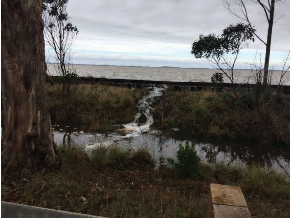
Photo 21 (approx. 2017): View facing west of flooding through damaged railroad prism (Segment 7).
