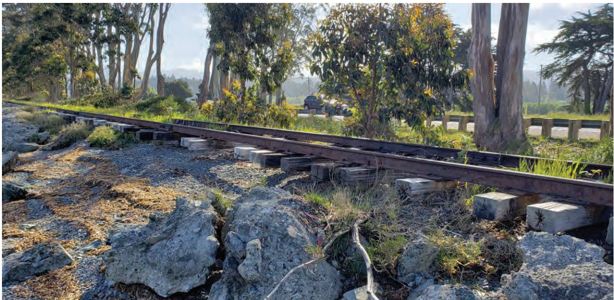
Photo 16 (May 2, 2019): View facing northeast of erosion of railroad prism (Segment 7).
