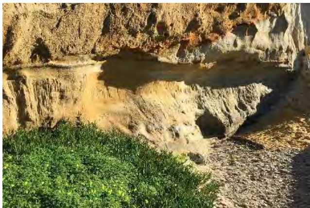
Photograph 1: Bluff Erosion and Overhang
