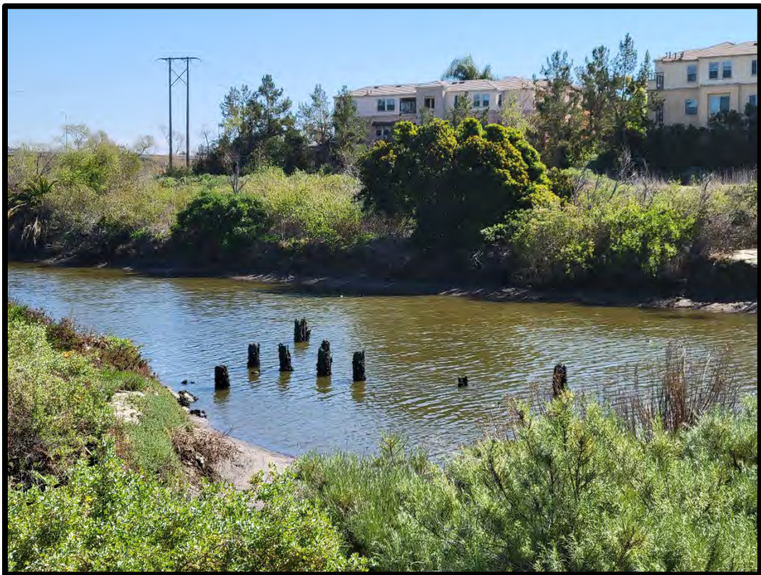
Derelict piles in San Diego Creek (eight visible and seven submerged.)
