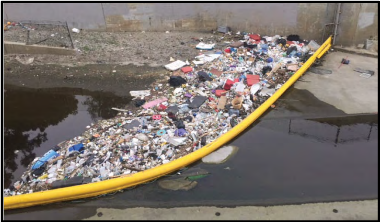
Boom installed in Santa Ana Delhi Channel.
