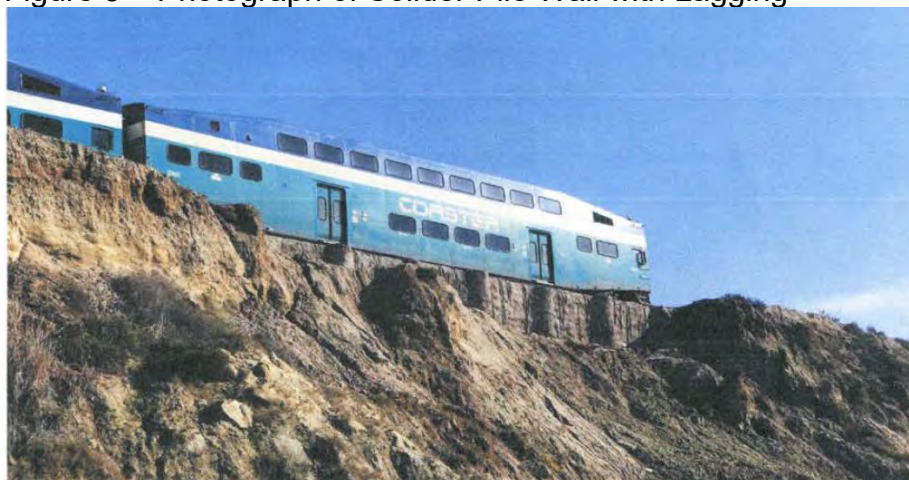
Figure 3 – Photograph of Soldier Pile Wall with Lagging
