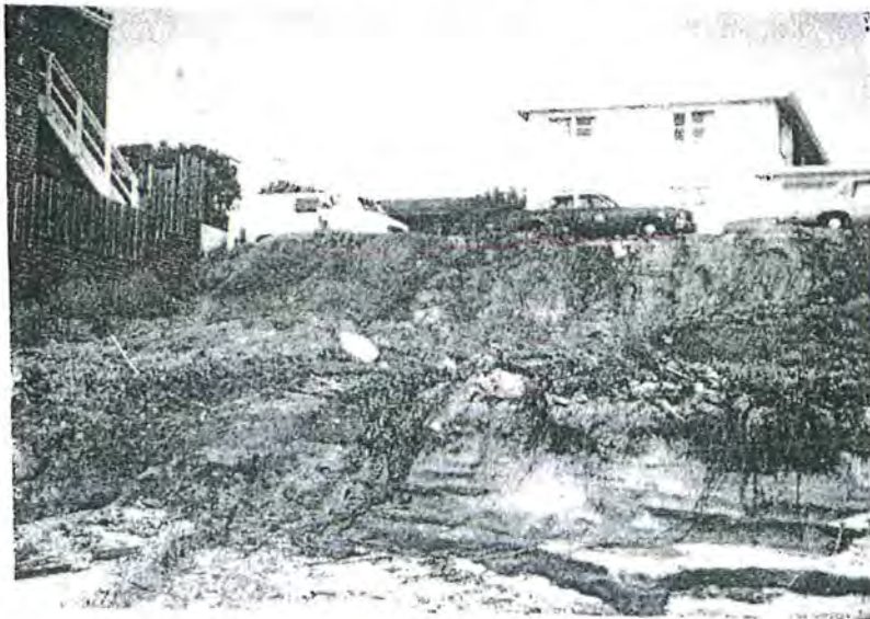
(b) Land erosion between Wisconsin and Hays Streets caused by wave action from the February 1980 storm.
