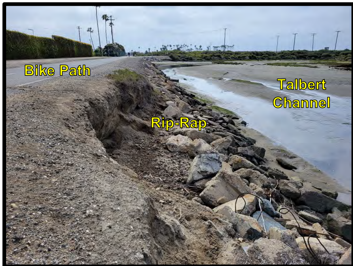
Figure 1. Portion of northeastern bank with sparse rip-rap and collapsed slope.
