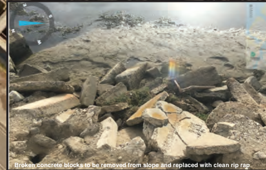
Broken concrete blocks to be removed from slope and replaced with clean rip rap.
