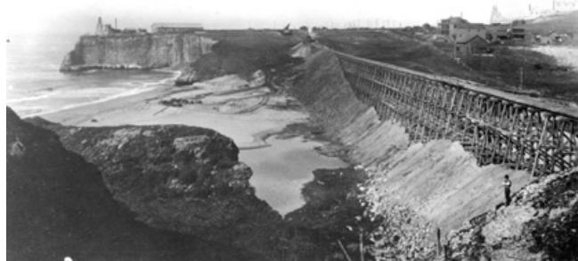
THE SAN VICENTE CREEK TRESTLE BEING FILLED IN, 1906.
