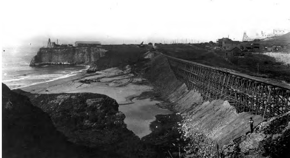
Figure 3: The historic rail trestle and fill at Davenport Beach. Photo: FHWA CD.
