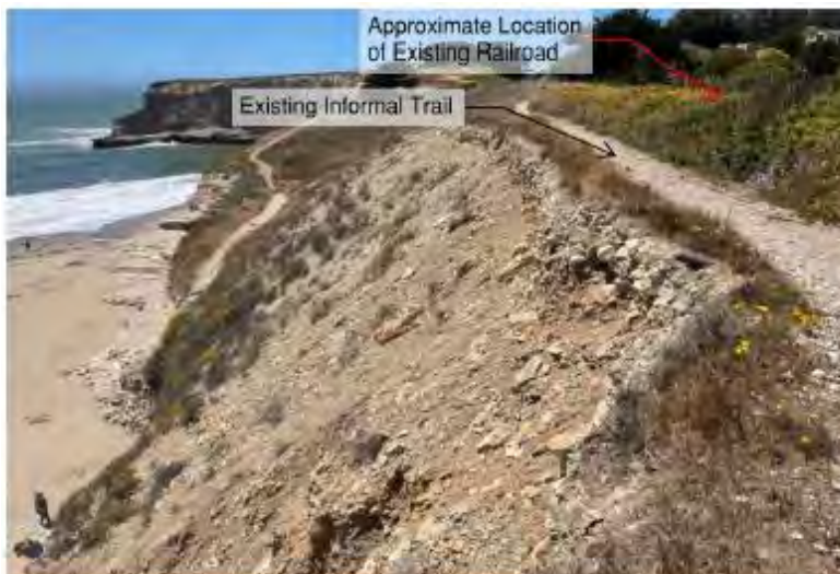
Figure 1: Informal trail and eroding slope. Photo: FHWA.
