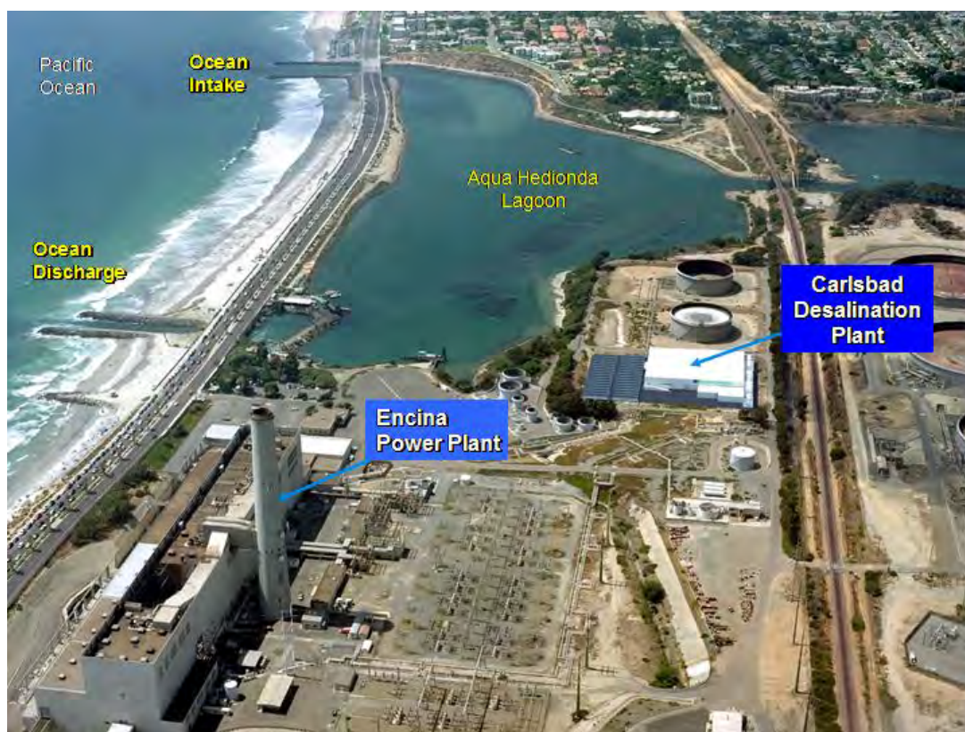
Figure 1 - Carlsbad Seawater Desalination Project
