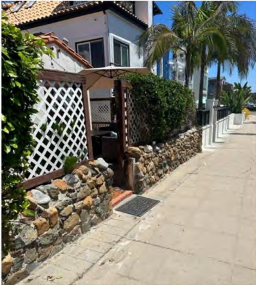
726 Jersey Court Frontage (looking east)
