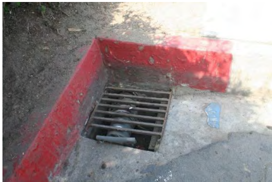
5. New pump inserted into the street and hidden inside the Beacons beach drain that travels to the Ocean. Note the blue NO DUMPING sign beside the drain has been chipped away.
