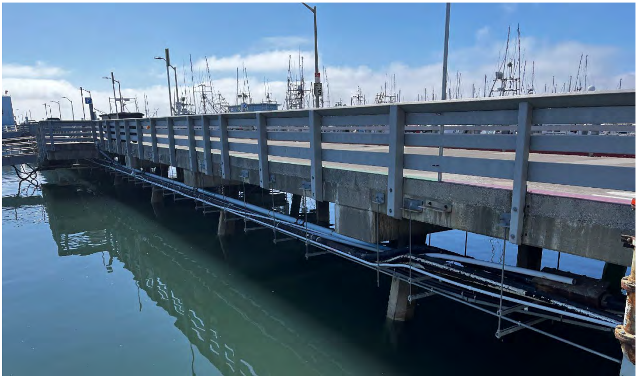
Figure 4. Utilities extending along pier trestle/stem.
