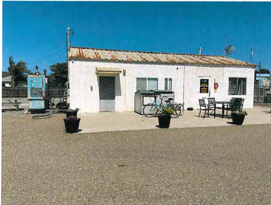
Figure 7: Pilot's Lounge Building (to be demolished and replaced with modular buildings)
