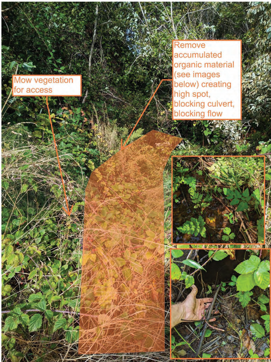
Photo 7. View east of vegetation blocking culvert between Peninsula Drive and Mill Street. Herbaceous vegetation would be mowed and debris removed from the channel.
