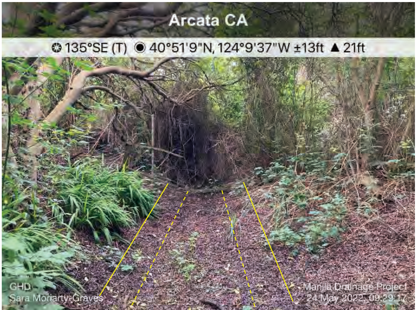
Photo 1. Area of temporary permanent one-parameter wetland impacts, three-parameter wetland impacts and wetland creation in the freshwater forested shrub wetland photographed May 24, 2022. Accumulated duff and vegetative debris the creates an elevation barrier to flow (see ponding created by barrier in Photo 2) would be removed between the dashed-yellow lines but the overstory would not be impacted. The channel here would be widened in the approximate area in between the solid-yellow lines and into the brush. Invasive Himalayan blackberry ( Rubus armeniacus ) would be removed and replanted with native vegetation. This location is the same as shown in Photo 2.
