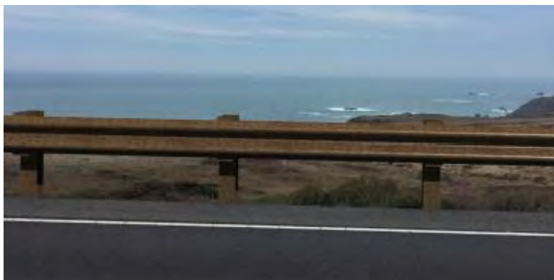
Proposed Midwest Guardrail System with light brown stain
