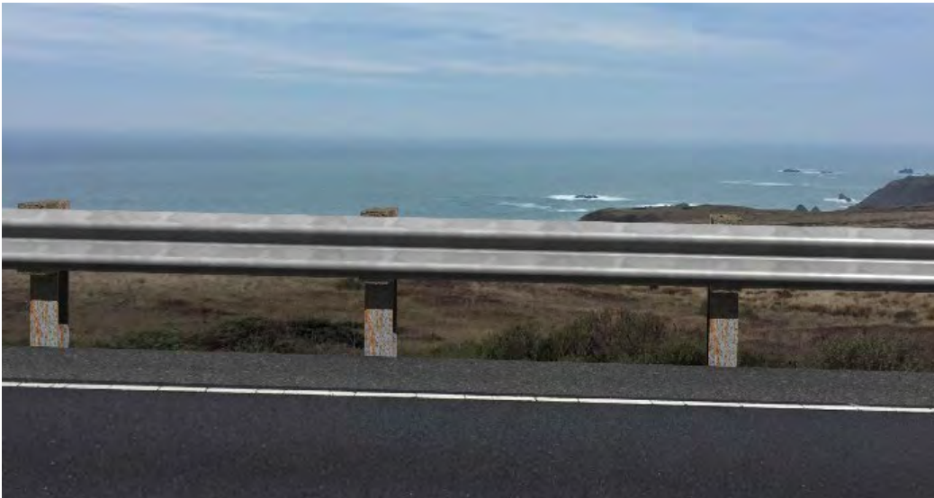
Figure 7 After MGS installation without staining.
