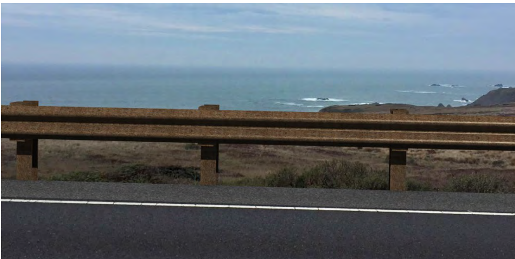
Figure 8 After MGS Installation without staining.
