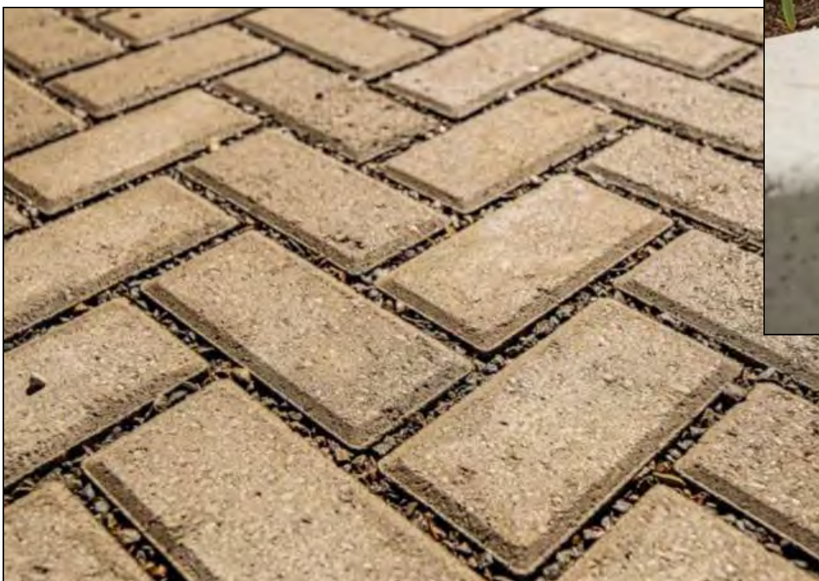
Porous pavers at parking and entry for stormwater control
