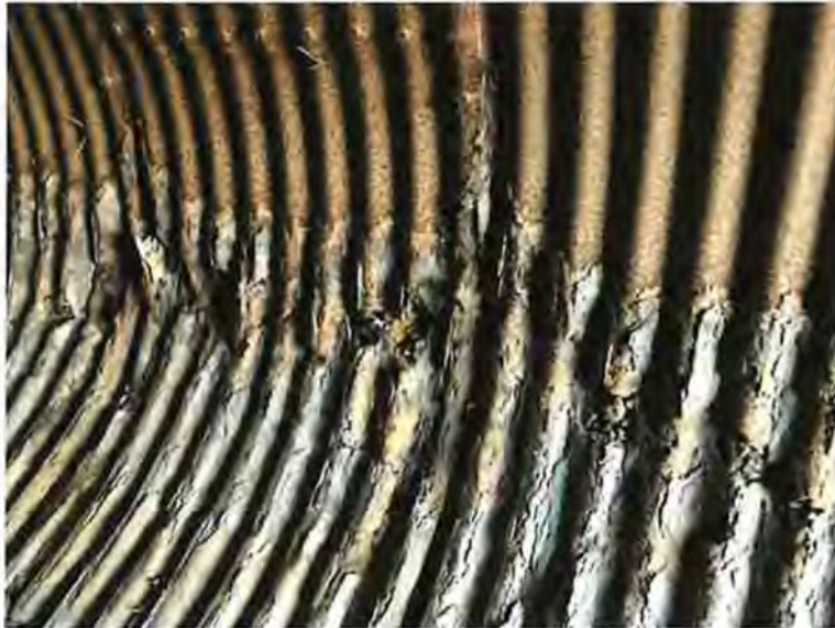
Damaged Culvert
