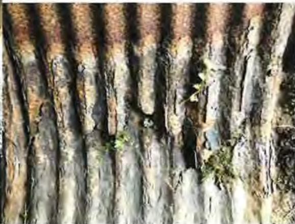
Damaged Culvert
