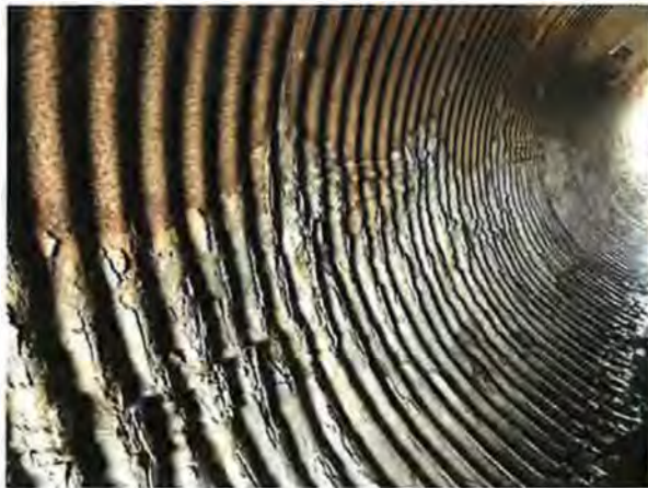
Damaged Culvert
