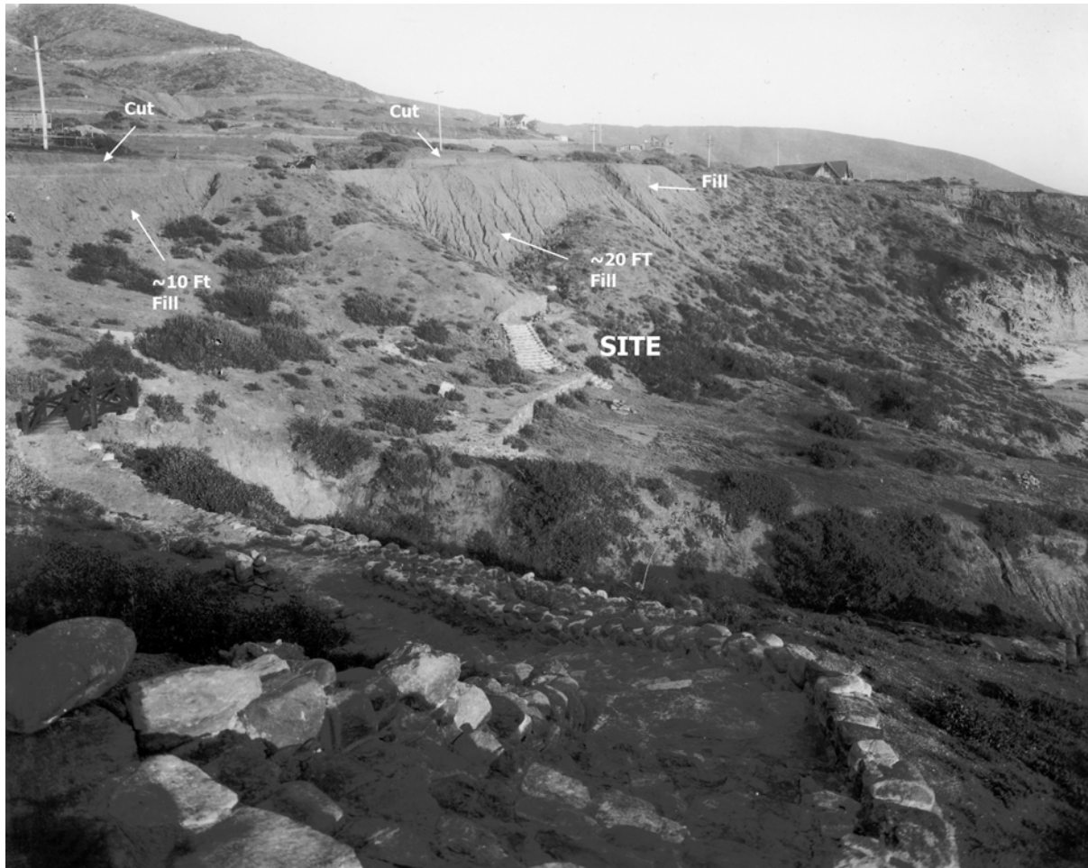
Figure 4 showing the extensive cut and fill grading that occurred at the site as a result of the construction of Coast Highway.
