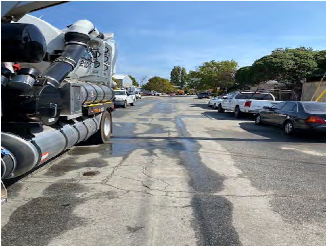
Vacuum truck capturing runoff
