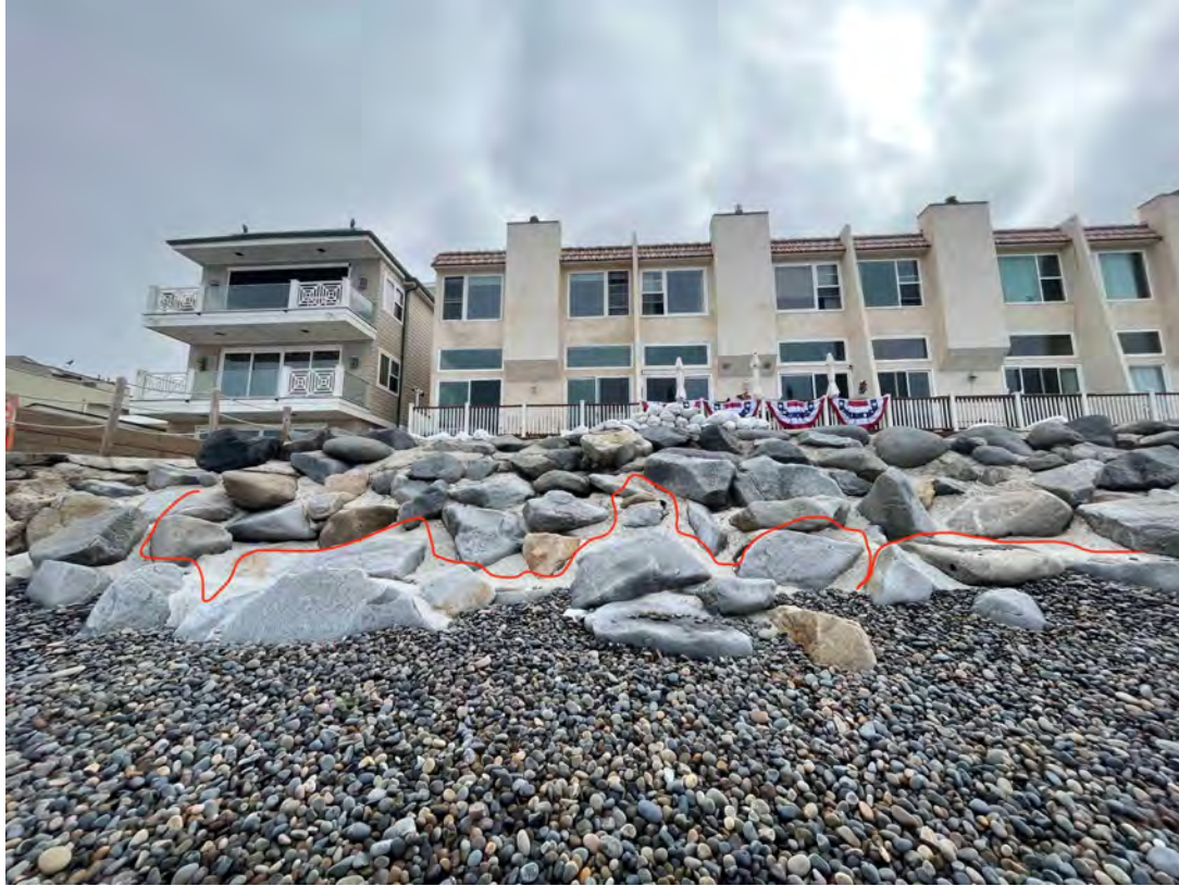
The red line traces concrete grouting
