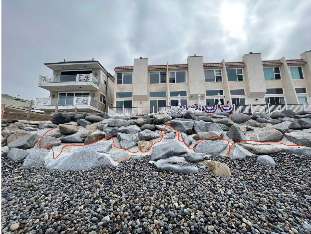
The red line traces concrete grouting
