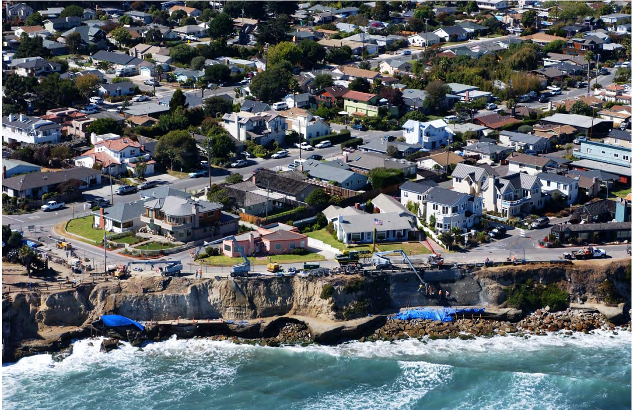
Figure 9. Construction of the tied-back wall east of Pleasure Point in 2004 (California Coastal Records Project).
