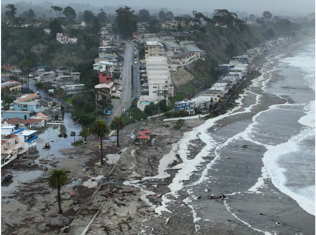
Figure 2 Rio Del Mar Flats and Beach Drive wave runup and flooding (Credit: Santa Cruz County Sheriff's Office)
