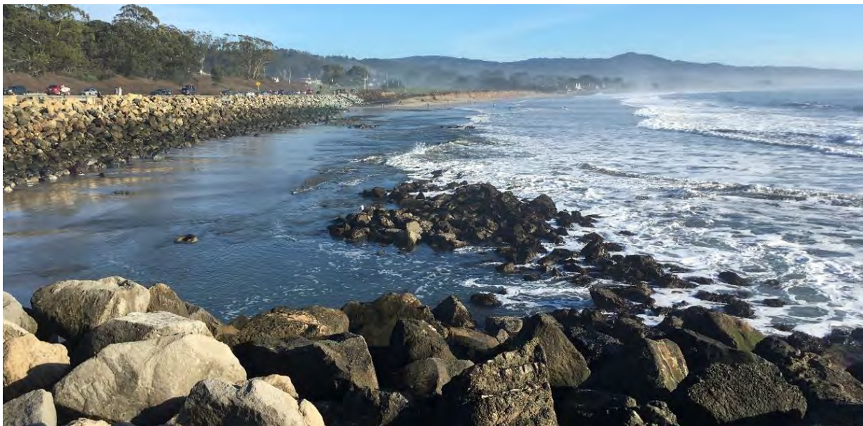
Figure 2. Photo of Surfers Beach on January 13, 2021, at low tide, showing Highway 1 at left with rock revetment, eroded beach and exposed rocks.
