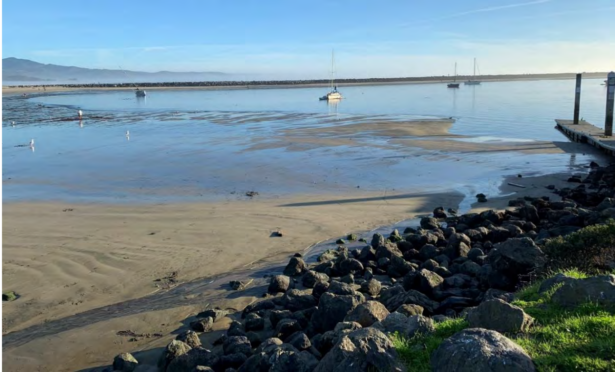
Figure 3. Photograph showing significant accumulation of sand near boat launch ramp in foreground and along the East Breakwater in background (1/13/21).
