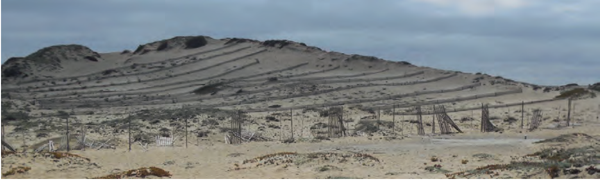
Figure 4-4: Multiple lines of wood slat fencing, oriented perpendicular to dominant onshore winds, was used in combination with jute netting to stabilize a wide artificial blowout in dunes at Marina, Monterey Bay. The lack of upwind sand supply from the coarse-grained beach allowed stabilization without formation of shadow dunes in lee of any of the fences. Note the vandalism and degeneration of the outer fenceline bordering public access. Interior fences are intact. April 2013.
