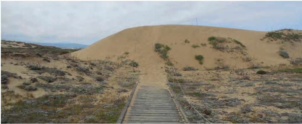
Figure 4-10: Active dune transgression over wood boardwalk, Marina Dunes State Park, Monterey Bay. Structural pedestrian walkways in mobile dunes are seldom stable, and rarely feasible to retrieve or rehabilitate after burial. April 2013.
