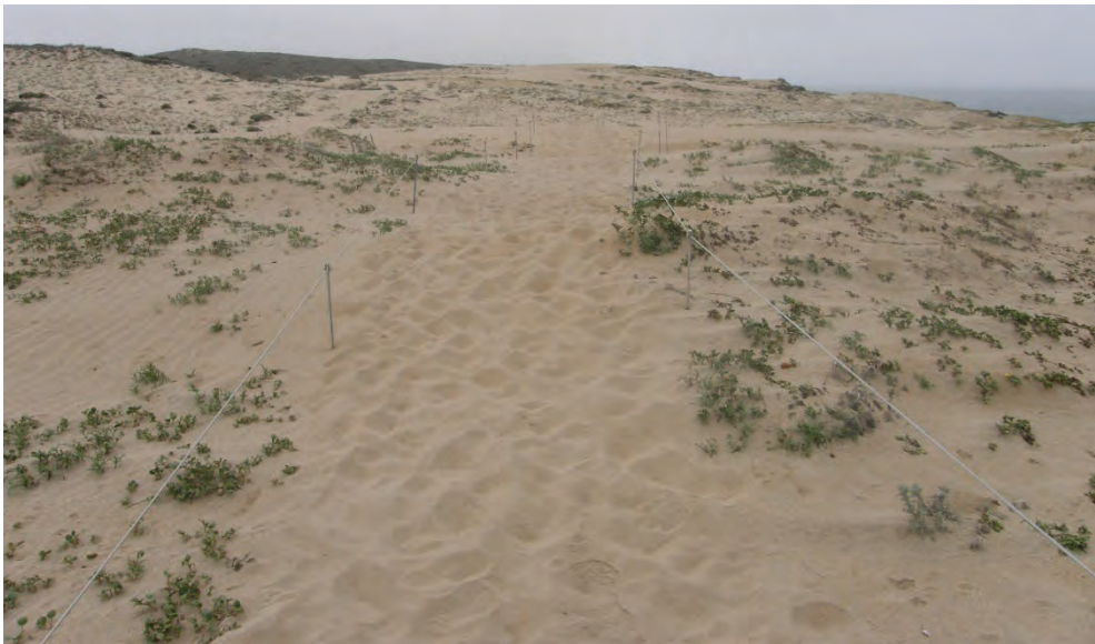
Figure 4-11: Symbolic cable fencing guides foot trails that are oriented perpendicular to dominant winds at Marina State Park, Monterey Bay. Cable fencing is transparent to eolian sand transport, erosion and deposition processes. Footprint patterns here indicate a high degree of compliance in conjunction with signage, despite ordinarily high visitor use. April 2009.
