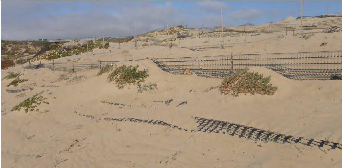
Figure 4-5: Plastic porous fences are used as less expensive substitutes for wood slat fencing, but are prone to breakage and vandalism, and are a high risk for debris (plastic pollution) on beaches. Sand City, Monterey Bay, 2009.
