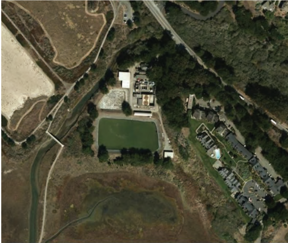
Bodega Bay PUD Wastewater Treatment Plant
