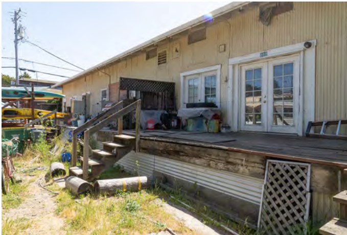
Figure 10: Oblique view of central portion of rear (north) façade. Looking southeast.
