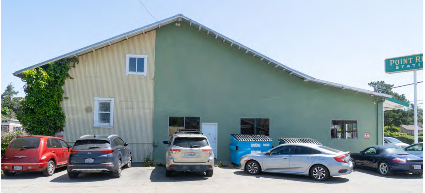
Figure 12: West façade of building, looking east.
