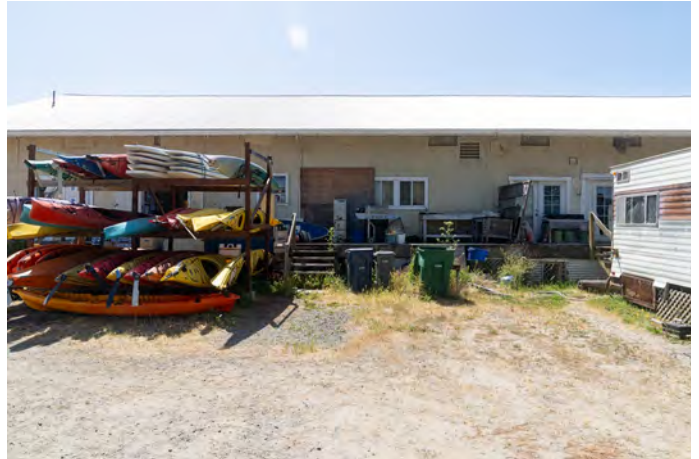
Figure 9: Central portion of rear (north) façade. Looking south.
