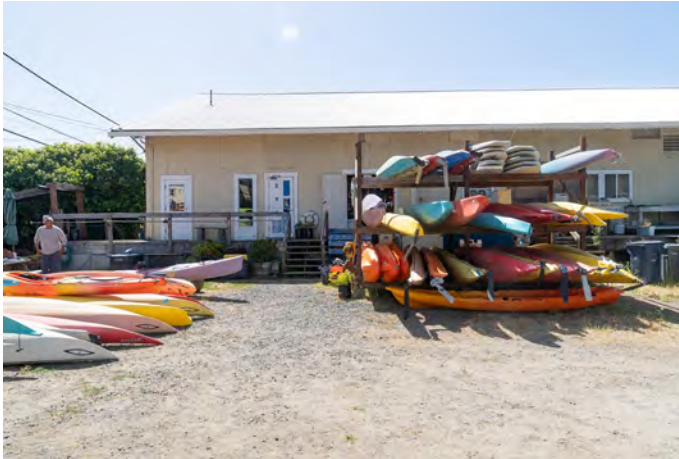
Figure 8: East end of rear (north) façade. Looking south.
