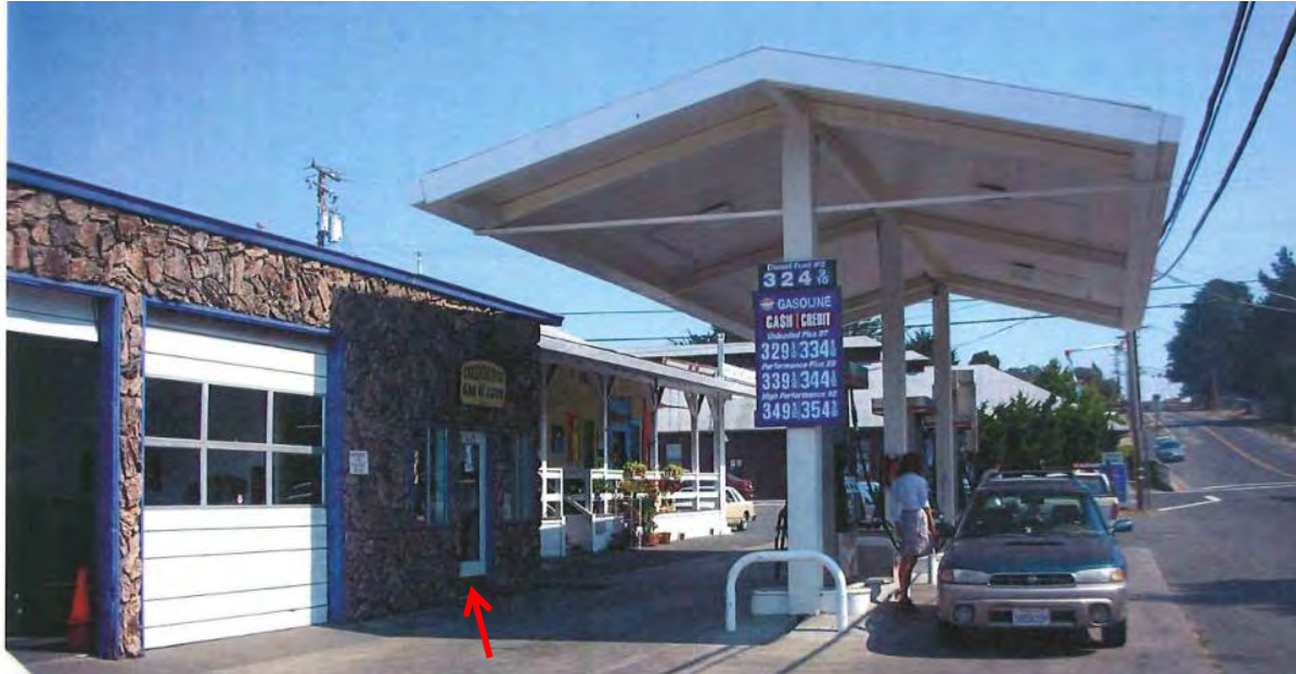
Figure 21: Subject building in 2007, showing faux stone cladding on primary façade and entry door location to commercial unit prior to its relocation and the replacement of this commercial unit's windows. Source: Marin County Building Department.
