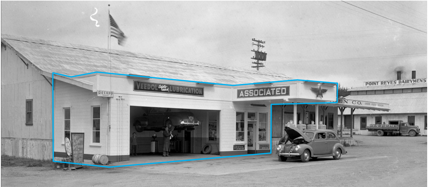
Figure 18: View of the primary façade of the subject building, looking northeast, circa 1948, showing the addition that housed a service station and gasoline station. Area outlined in blue shows area of addition. Source: Jack Mason Museum of West Marin History.
