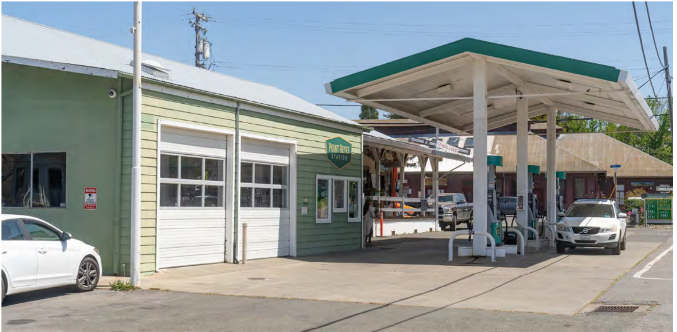
Figure 1: Oblique view of primary façade showing addition at west end of the façade. Looking northeast.
