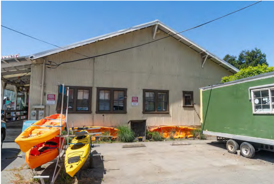
Figure 6: East façade, looking west.
