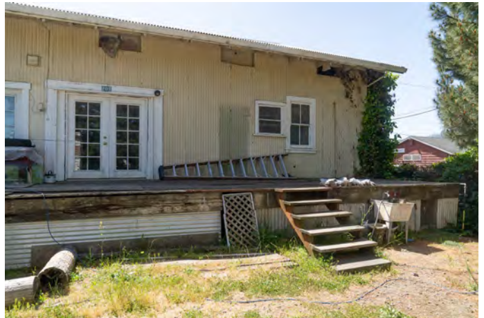
Figure 11: West end of rear (north) façade. Looking slightly southwest.
