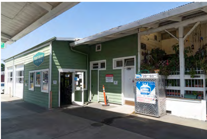
Figure 2: Oblique view of primary façade, looking northwest.
