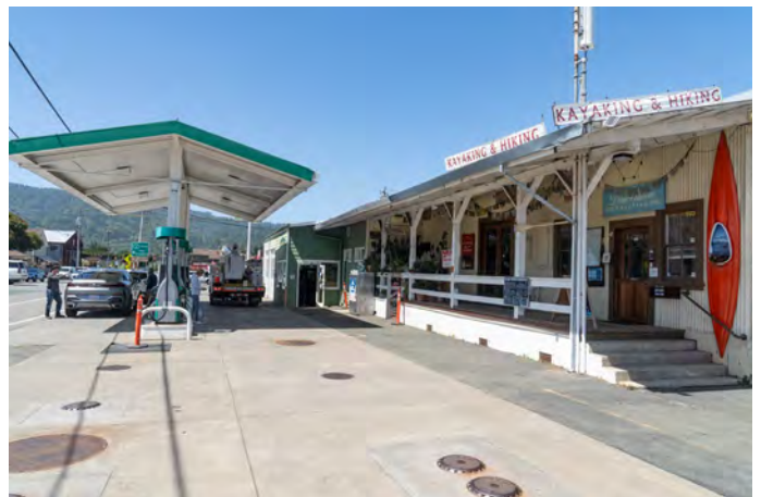
Figure 3: Oblique view of primary façade as seen from east end of building, looking northwest.
