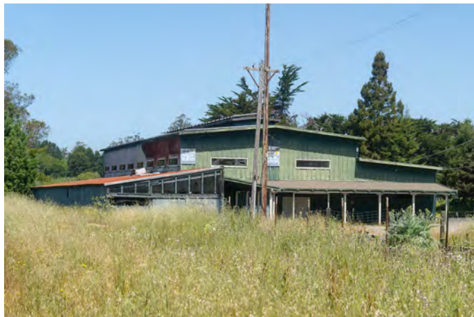
Figure 16: Old railroad barn at 510 Mesa Road, built ca. 1920.
