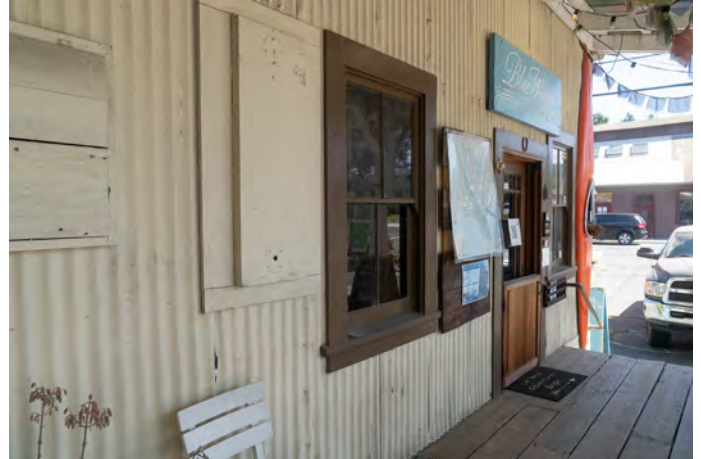
Figure 5: Openings at east end of covered porch, looking northeast.
