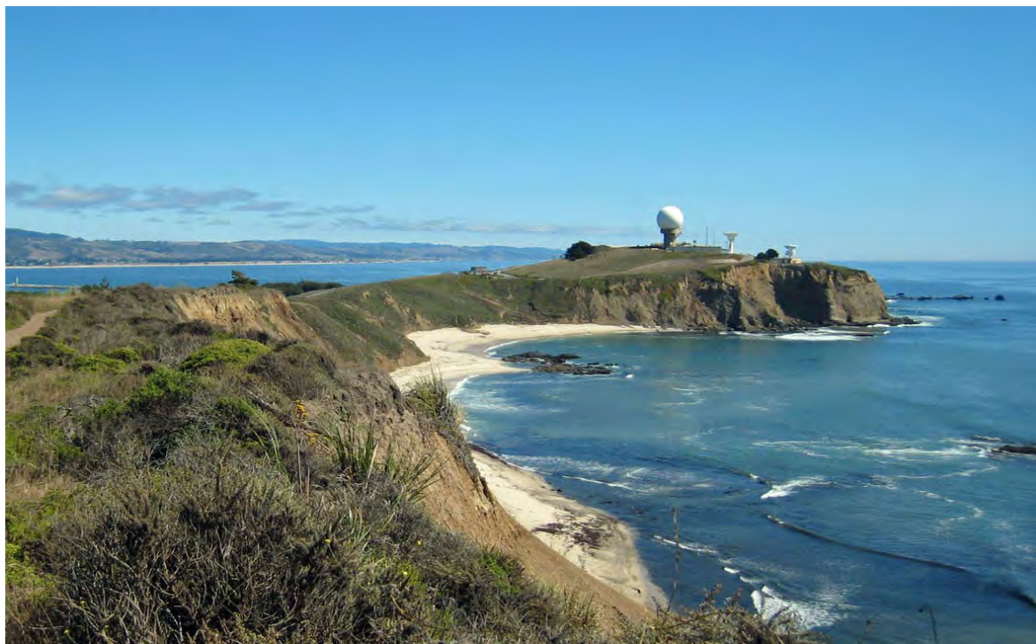
Figure 7a. Current view of PPSFS from public trail north of the site looking back towards Ross' Cove. Photo credit: Lisa Ketcham
