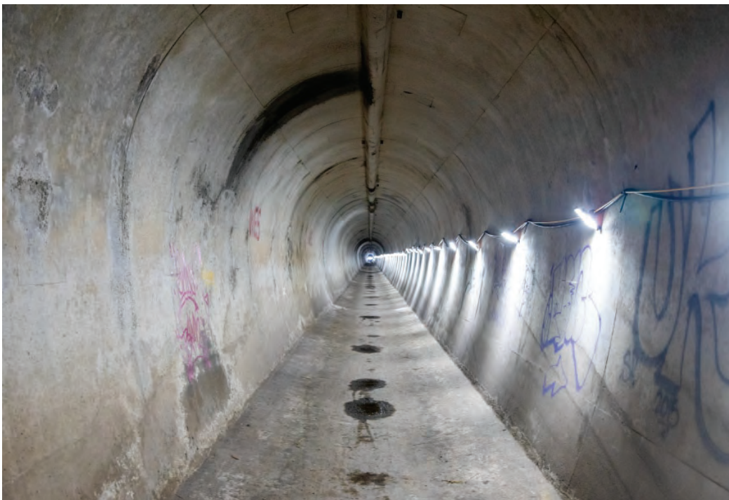
Lake Merced Tunnel 14'0" in diameter
