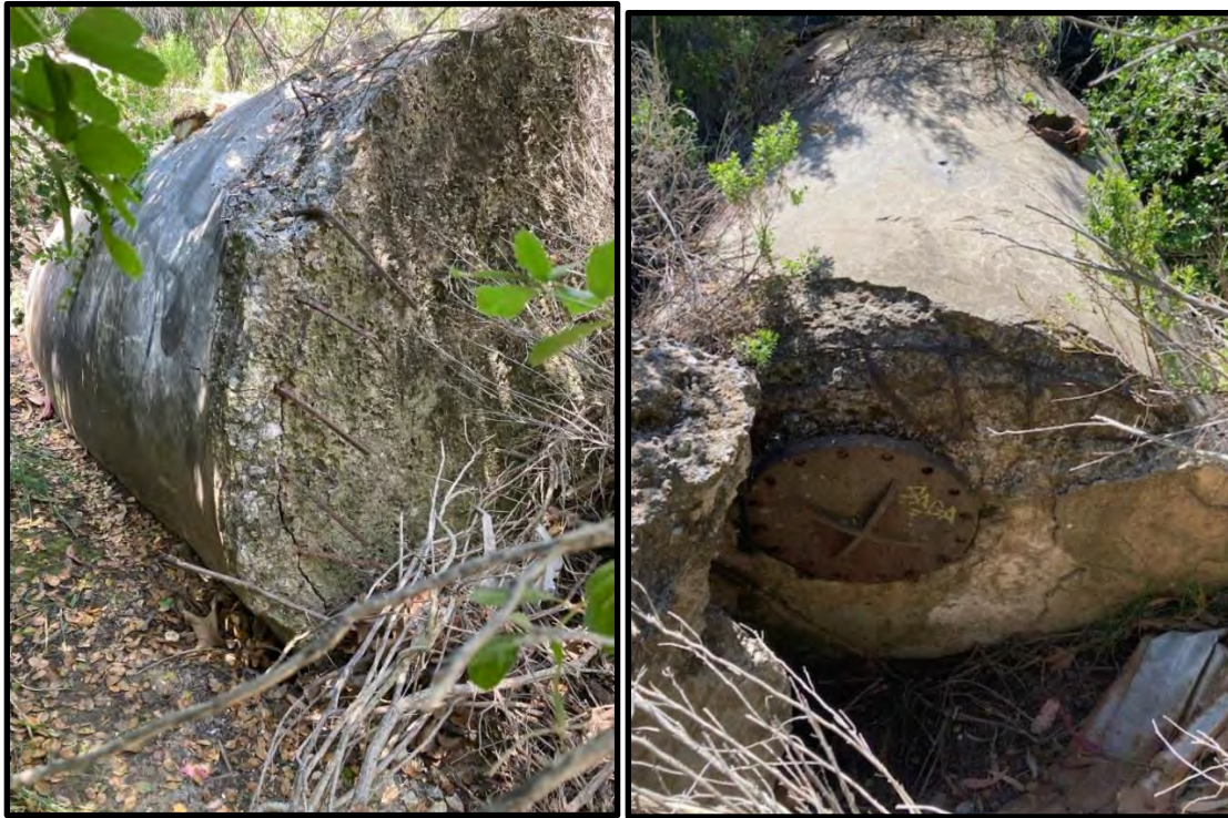
Figures 4 and 5-Discarded Underground storage tank. Note fill port and graffiti marked access hatch on the UST.
