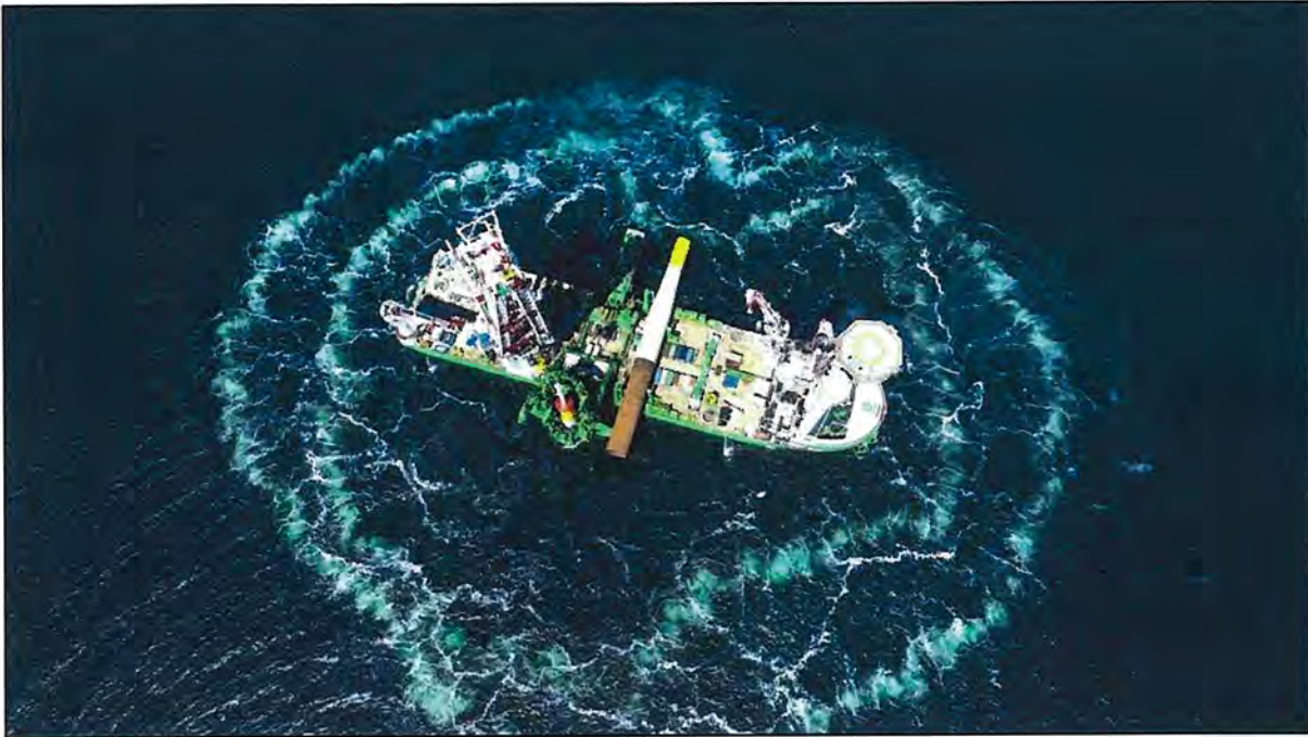
Figure 2. Drone view of the Orion showing double bubble curtains operating. Air compressor support vessel is out of frame at lower left edge of photo. The hydro sound damper is hung around the monopile from sea level to seabed. Photo by DEME [7].
