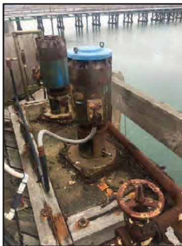
Image 2: Existing water intake pumps at the Redwood Marine Terminal II Dock. These will be replaced.
