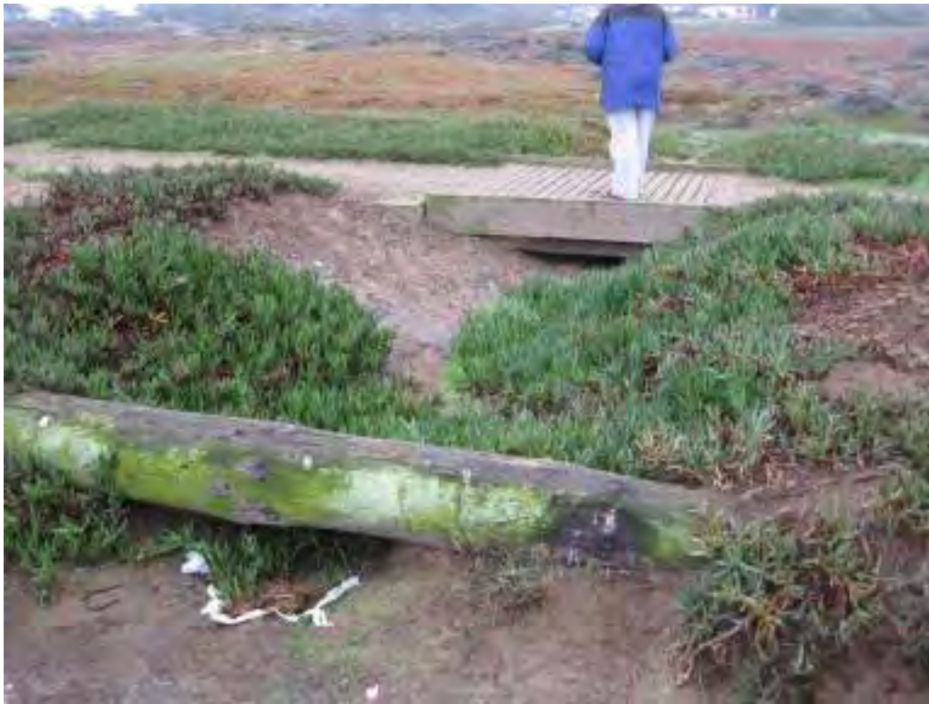
Photo 3: Vegetated swale at Fort Funston collects parking lot runoff (11/07/12)
