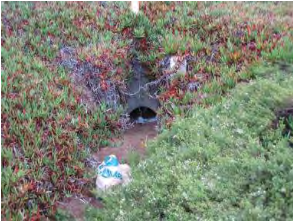
Photo 4: Downstream end of vegetated swale, which discharges into culvert and sewer system (11/07/12)
