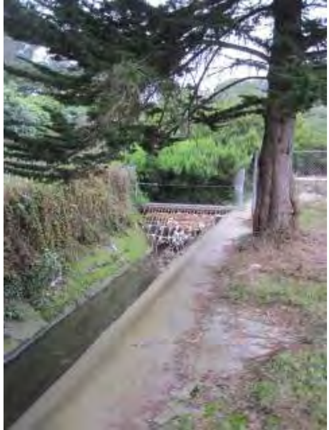
Photo 8: Downstream end of Vista Grande Canal, with trash rack and tunnel entry (11/07/12)
