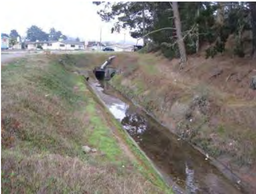
Photo 5: Upstream end of Vista Grande Canal shows typical wide reach of canal with OHWM of 11.5 feet (11/07/12)
