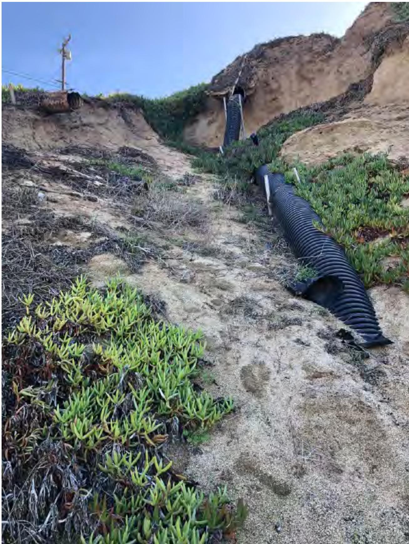
Existing Condition: Exposed Broken Corrugated Metal Pipe with Temporary Pipe in Place in Eroded Gully
