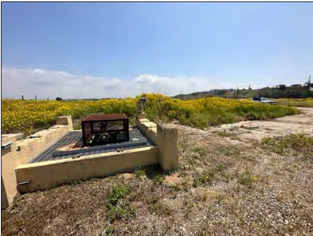
Photo B-2: DR-4 overview. Photo facing east.
