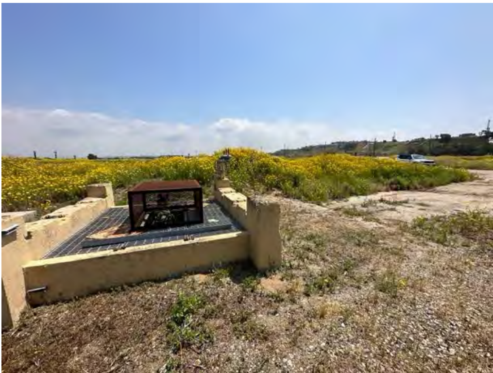
Photo B-2: DR-4 overview. Photo facing east.
