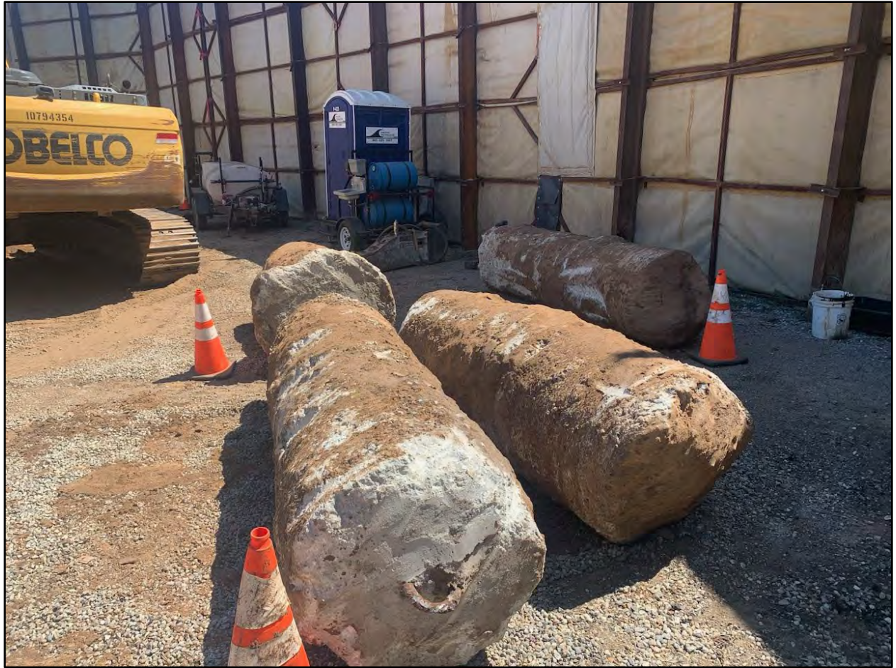
Figure 4. Rig Anchors pulled from SoCalGas' Harper 1 well site.
