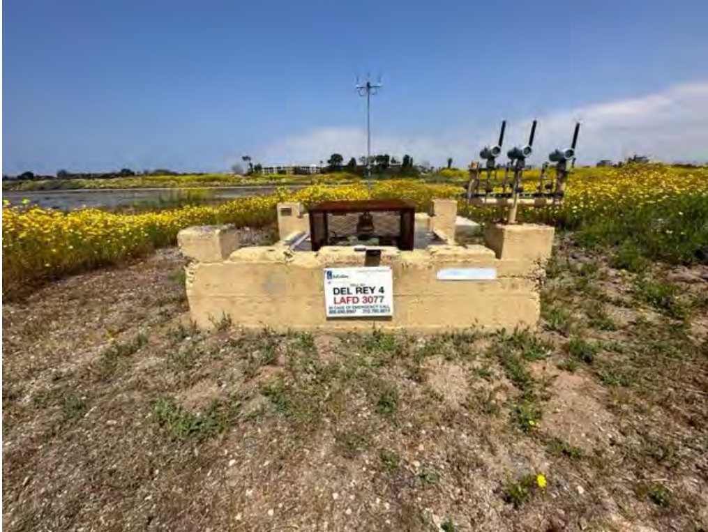
Photo B-1: DR-4. Photo facing northwest.
