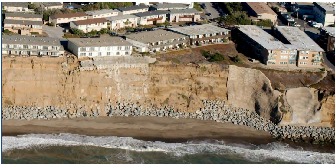
Figure 8. Photo of Esplanade Apartments threatened by cliff erosion in 2013 in Pacifica, CA. (Source: California Coastal Records Project )
