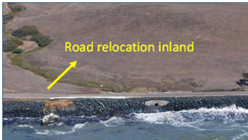
Figure 25. Photo depicting planned retreat for major public infrastructure. The Piedras Blancas Highway 1 Realignment will move nearly 3 miles (5km) of Highway 1 500 ft (152 m) inland. (Source: California Coastal Records Project )
