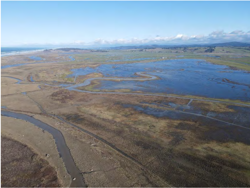
Photo 3—Drone footage from December 2021, looking northwest at the large interior slough channel (unnamed) that extends eastward into the Project Area, and another smaller slough channel that runs south. The existing levee system (and areas that have failed and breached), can be seen in the distant northern portion where there are small slivers of dry land.
