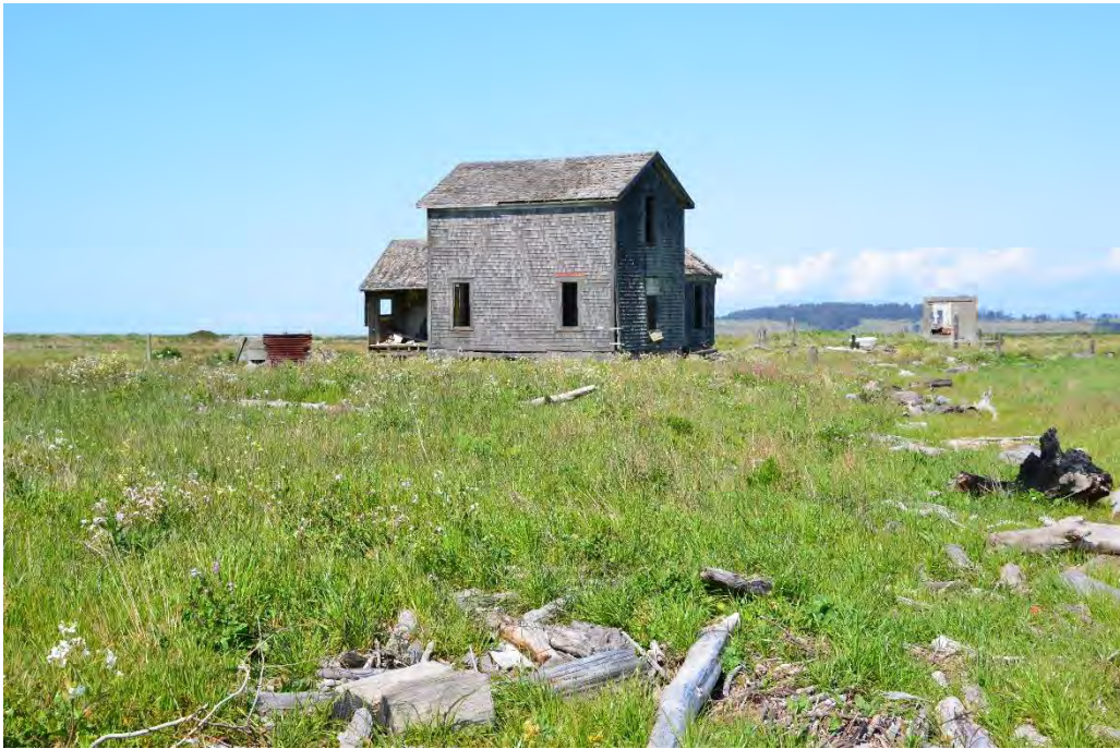
Photo 19—View of abandoned residential structure that is proposed to be demolished and removed from the non-native dominated ruderal habitat it was constructed in. This area will be reclaimed by full tidal influenced coastal salt and brackish marsh once the existing levees are graded to lower elevations.
