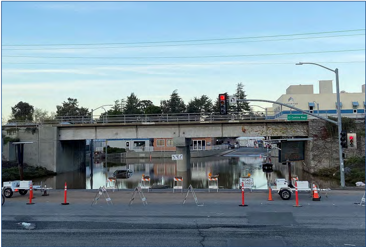
Figure B-8. Photo of pluvial flooding at an undercrossing in San Mateo, CA (Source: B. Washburn, www.flicker.com/btwashburn ; CCA 2.0)
