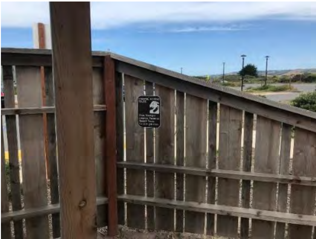
Figure 11. Signage installed at Overlook A (close-up).
